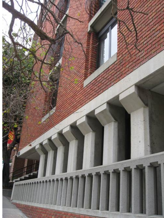
Detail of balustrade, looking northwest. (Page & Turnbull, March 2013)
