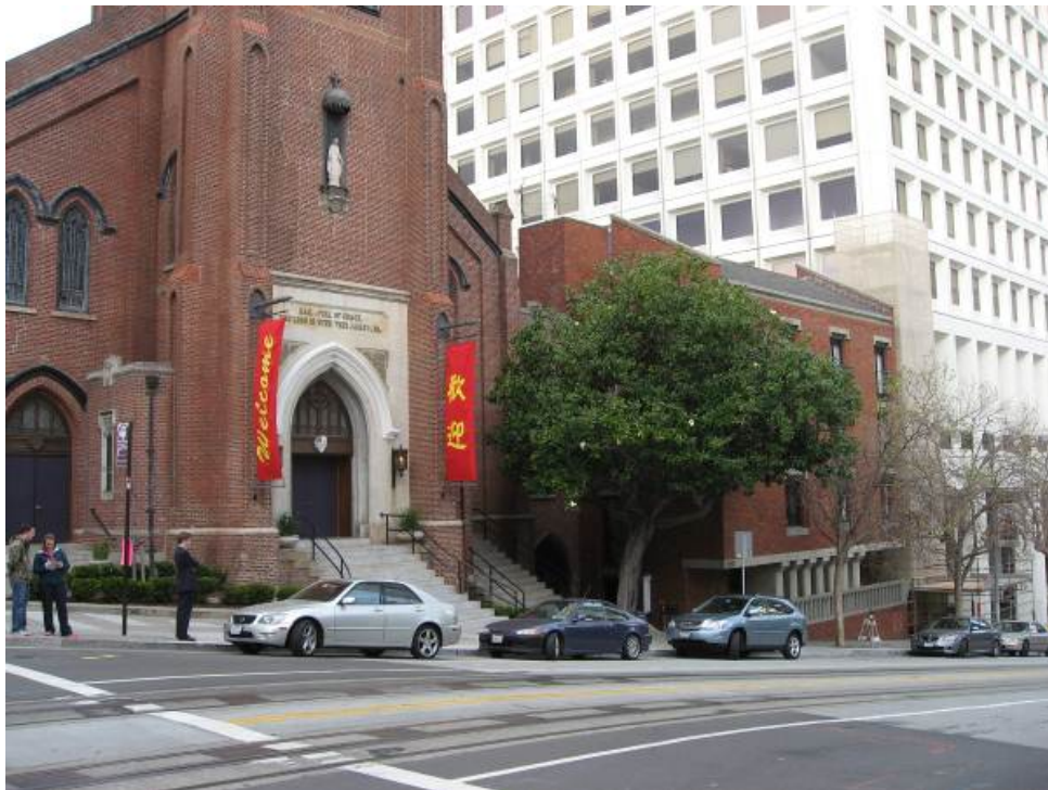
View northeast with Old St. Mary's at left, looking northeast. (Page & Turnbull, March 2013)
