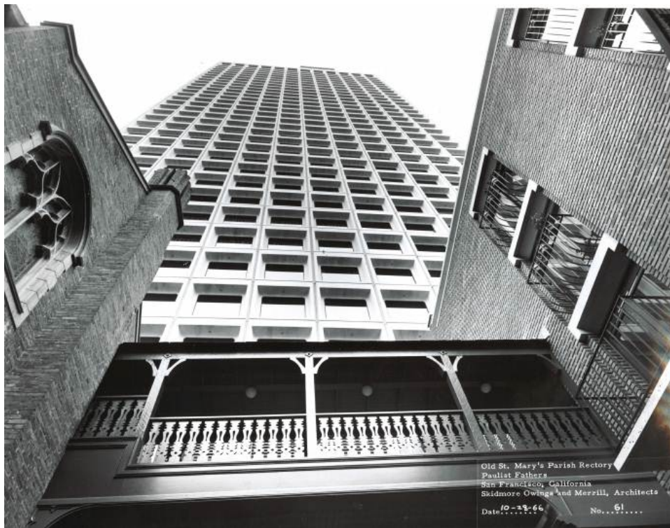
View showing the Sacristy (left), bridge and rectory (right) in relation to the Hartford Building, October 1966. (©Skidmore, Owings & Merrill LLP 2013)
