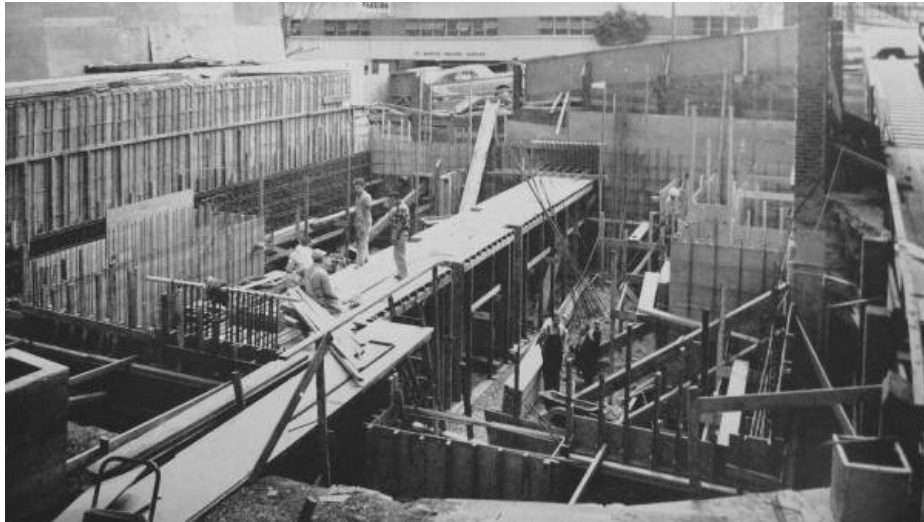
Construction of the new Rectory, 1965. (Paulist Calendar, November 1965.)
