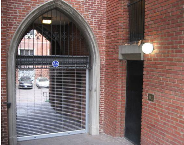
Detail of entry on west façade, adjacent to the bridge and gate to the rear parking area, looking northeast. (Page & Turnbull, March 2013)
