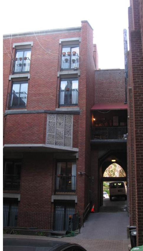
Detail of the west end of the rear (north) façade, looking south. (Page & Turnbull, April 2013)
