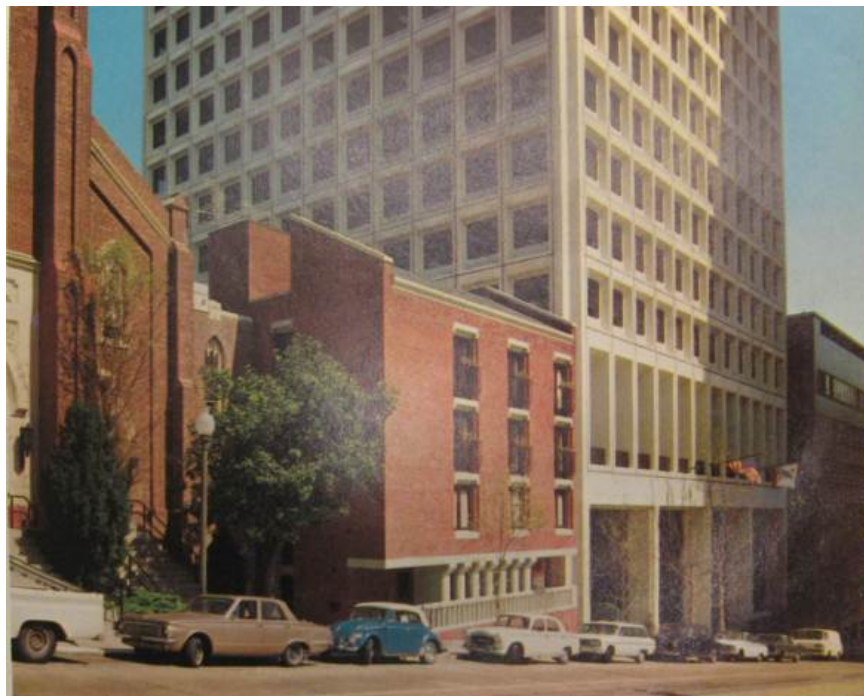
Old St. Mary’s Rectory and Hartford building. (Architectural Record, May, 1967, p.137)
