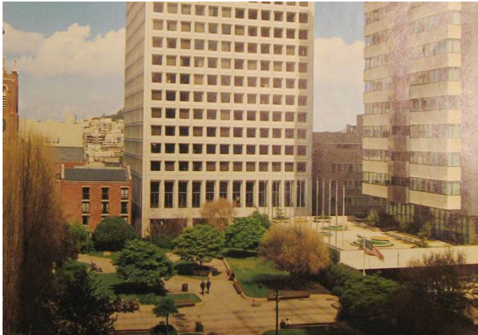
Old St. Mary's Rectory and Hartford building. (Architectural Record, May, 1967, p.131)
