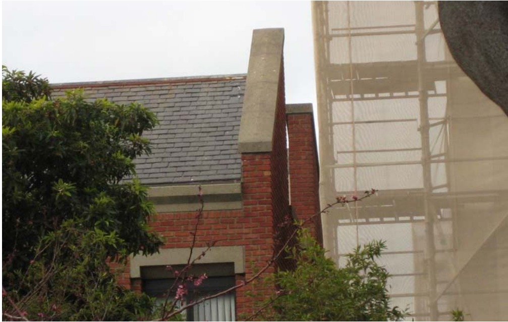
East façade, looking north from California Street. (Page & Turnbull, April 2013)
