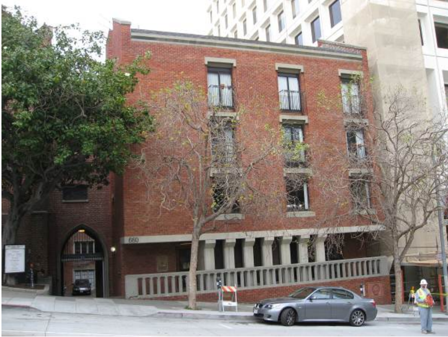
View north of the primary façade, looking northeast from across California Street. (Page & Turnbull, March 2013)
