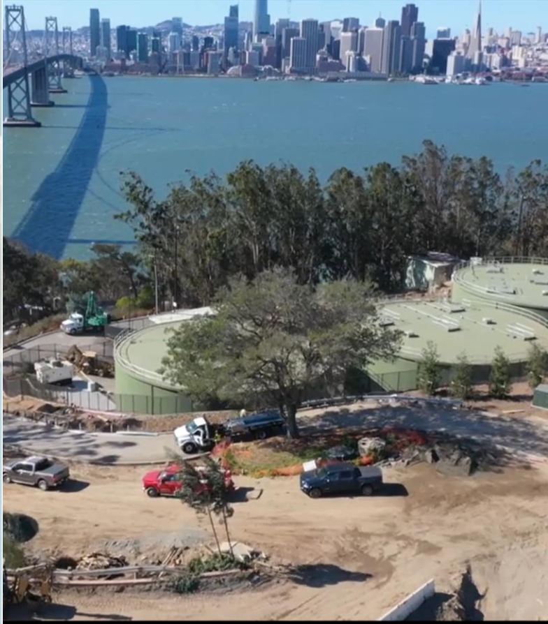
new water tanks
