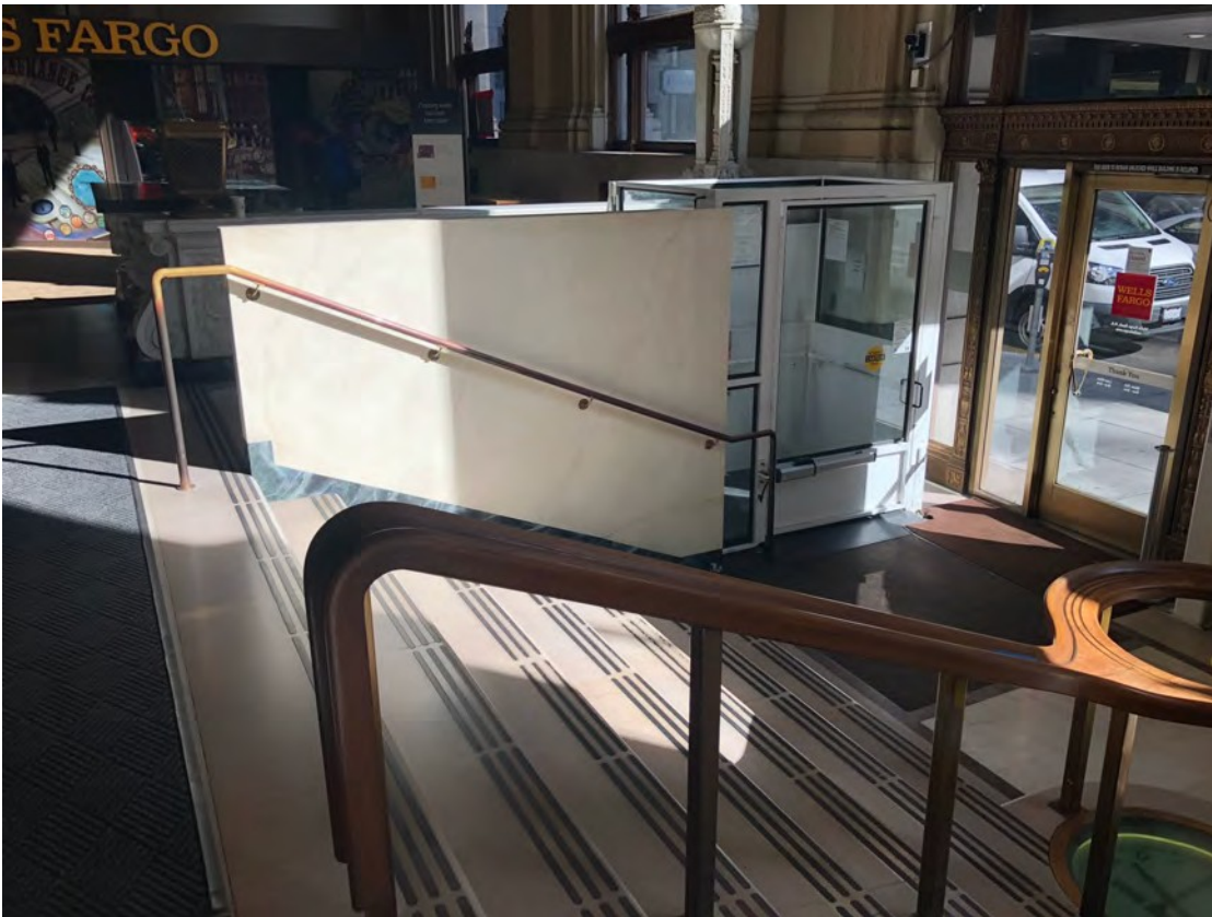
View of the Montgomery Street entry with the inserted lift and detail of railing, October 2019. Source: architecture + history, llc. (2020) report
