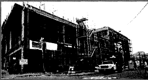
School Building Construction A Work in Progress as of Sept. 10, 2014
