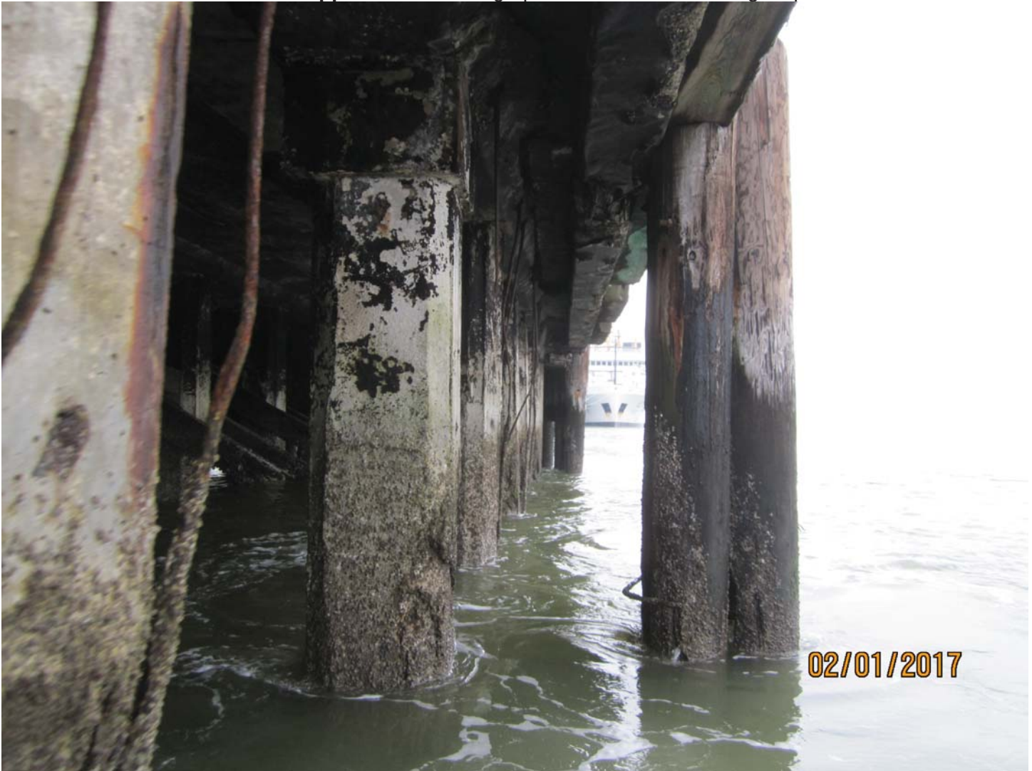
Photo 11. Concrete pile jackets along eastern edge of pier (looking north)
