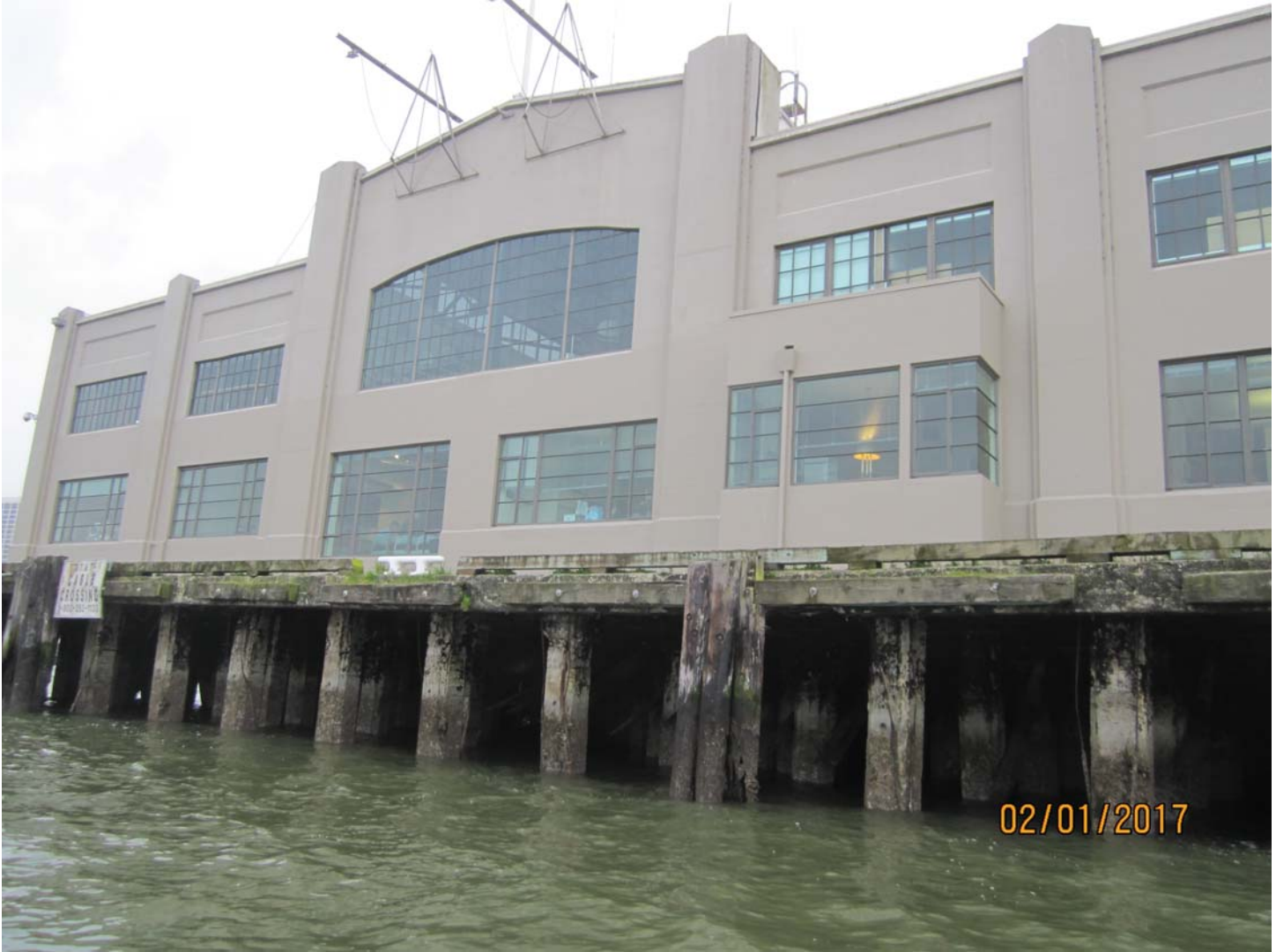
Photo 1. Outer end of pier
