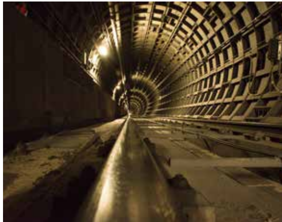
Muni Metro Tunnel
