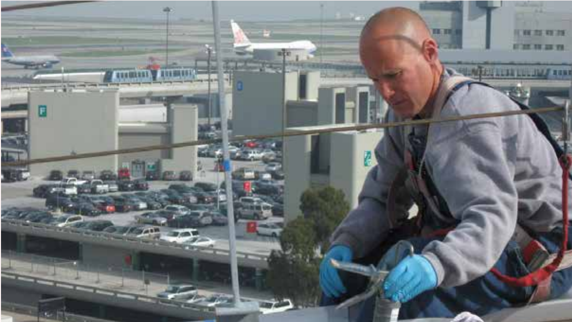
Roof Repair at SFO
