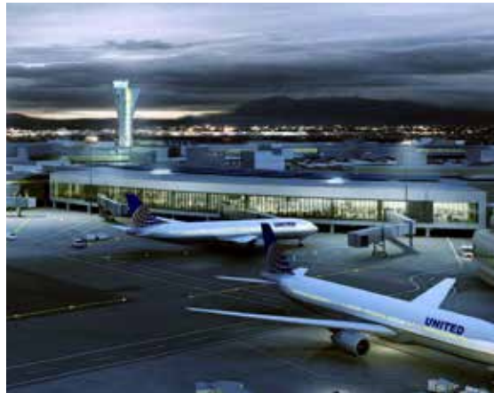
SFO Terminal 3 East
