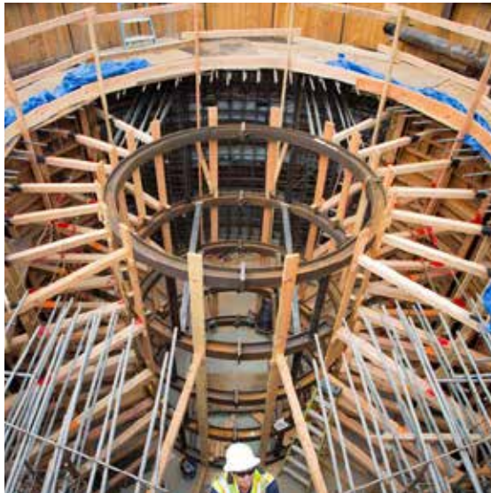
Water System Facilities Improvements
