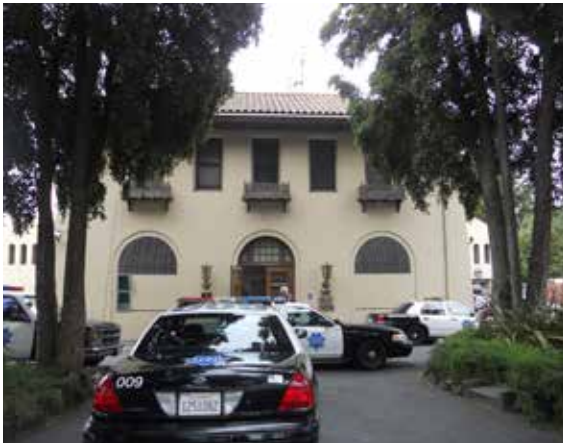
SFPD Park Station
