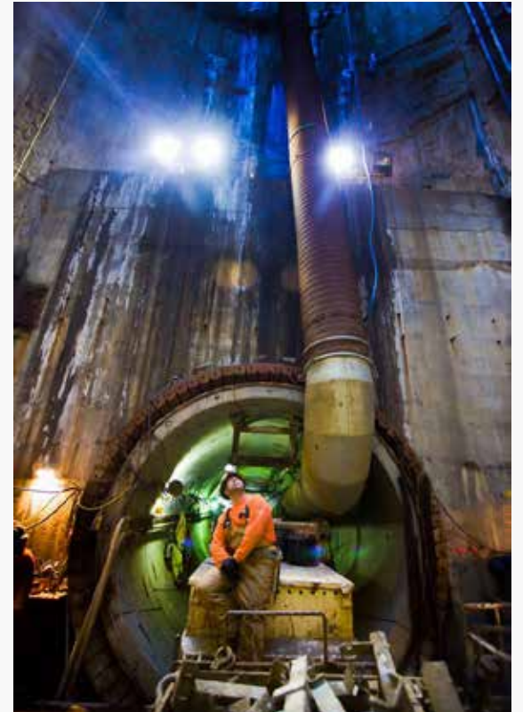
Ongoing Water Sewer Improvement Program
