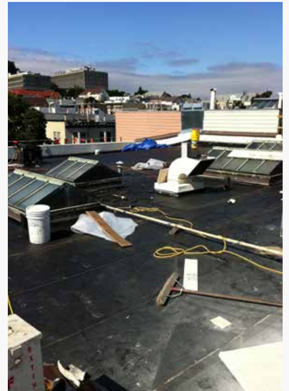
Roof Replacement at Fire Station 6
