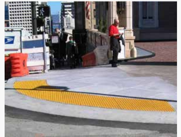
Newly Installed Curb Ramp
