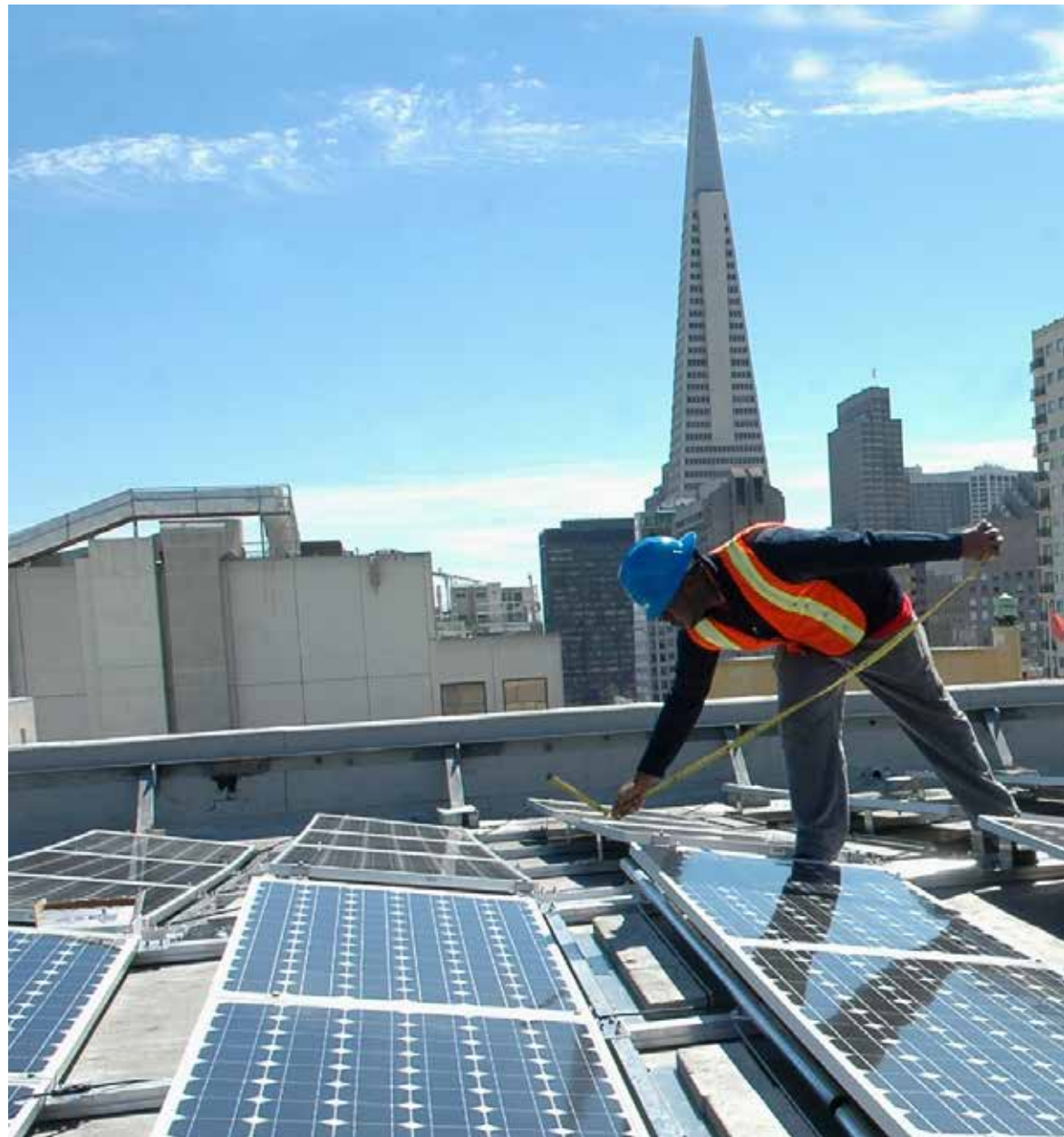
Solar Panel Installation at City Facilities
