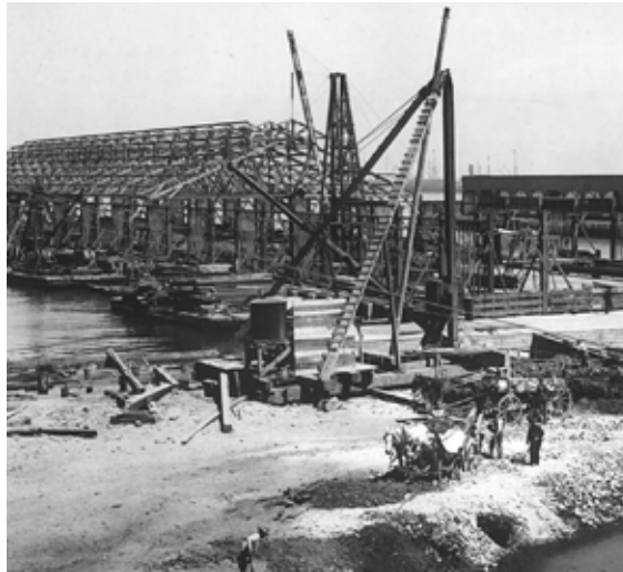
Construction of the Seawall
