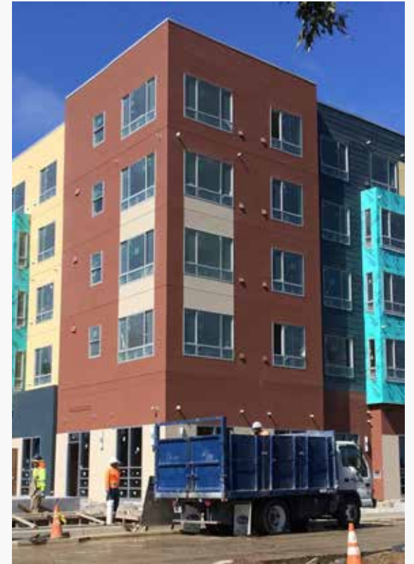
Construction at HOPE SF Alice Griffith
