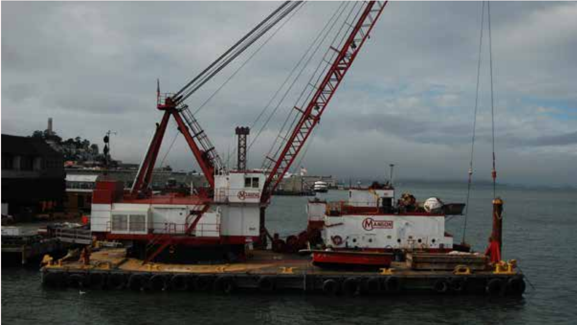
Dredging at the Port
