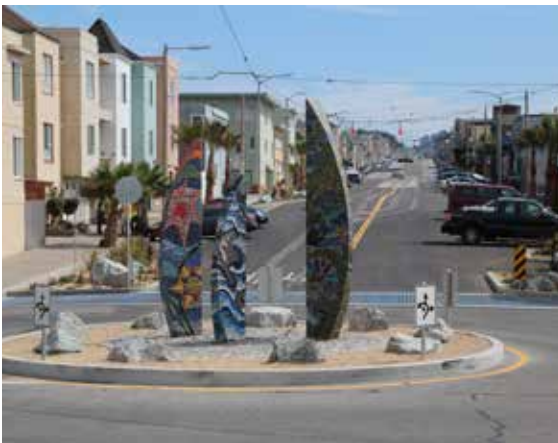
Recently Completed Taraval Streetscape Project
