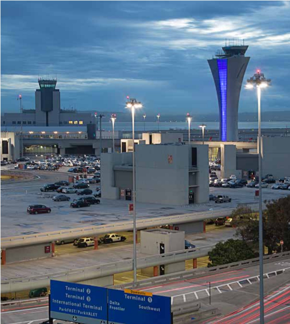
New Control Tower at SFO
