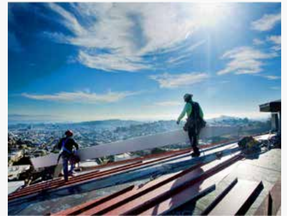
New Roof at the Ashbury Tank
