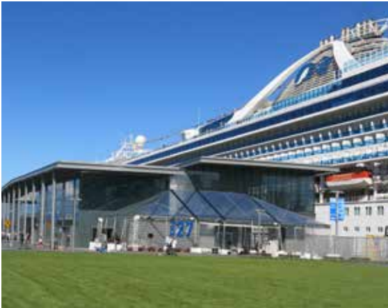
New Cruise Ship Terminal at Pier 27
