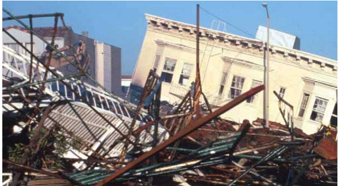
1989 Loma Prieta Earthquake
