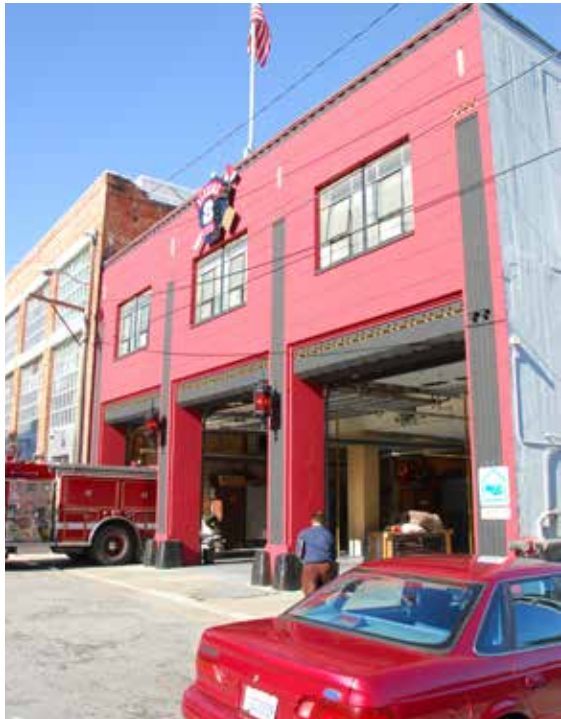
SFFD Fire Station
