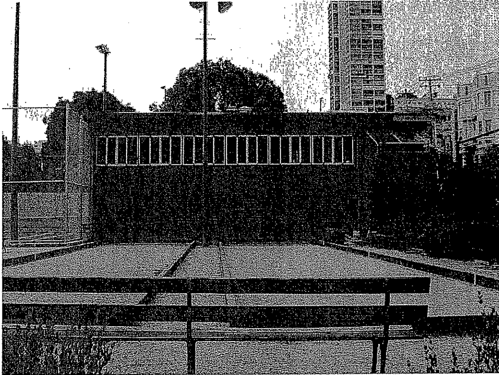
North Elevation of the North Beach Branch Library
