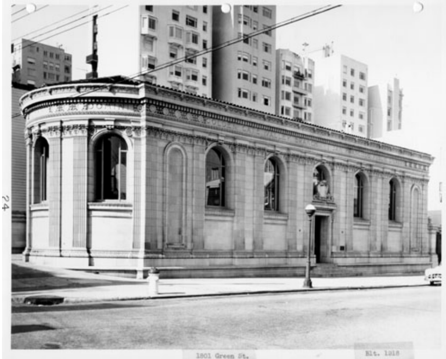
Above: Golden Gate Valley Branch Library, looking southwest. (Source: SFPL Photograph Collection, #AAC-5676).
