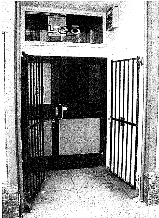
Figure 1. Metal entry door at west elevation.
