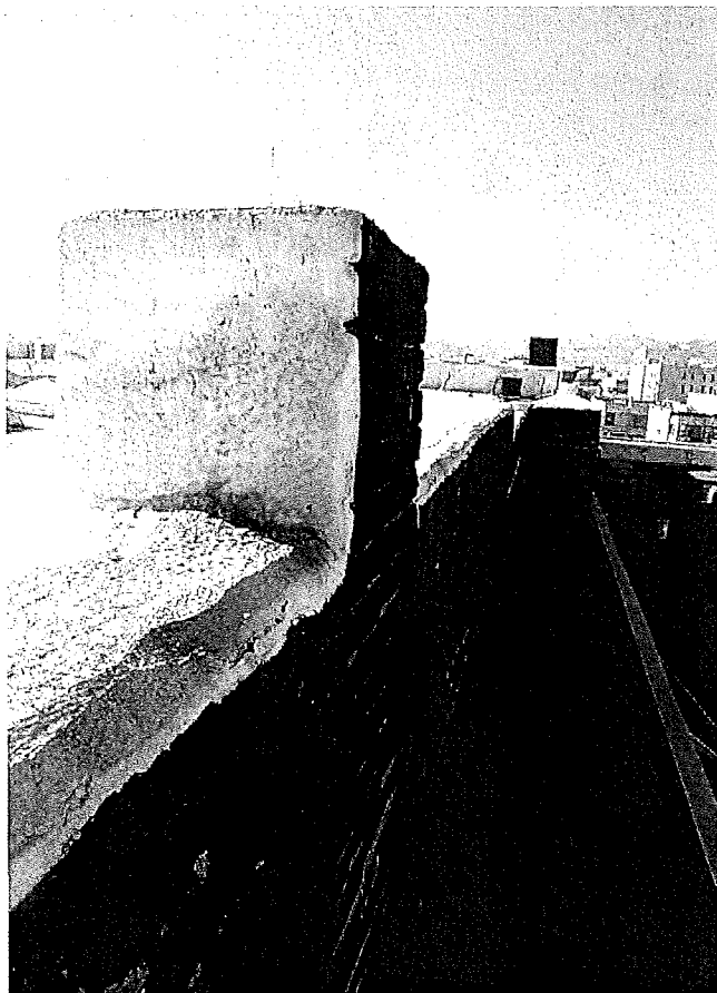
Figure 3. Unbraced ventilation stack at north wall.
