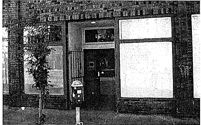
Figure 1. Storefront at west elevation.
