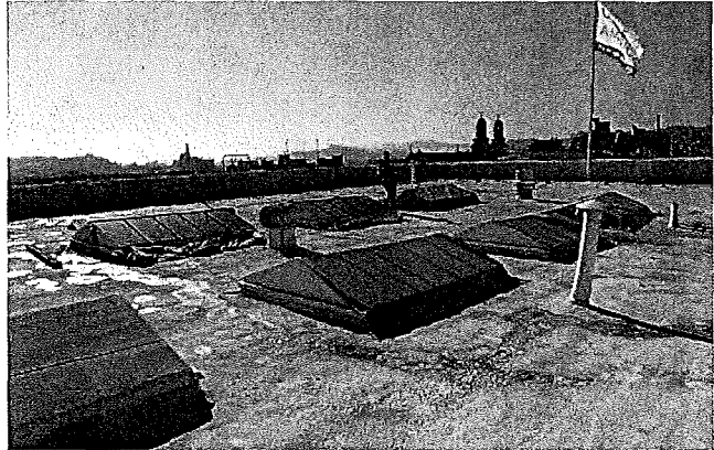
Figure 1. Roof overview; note skylights.
