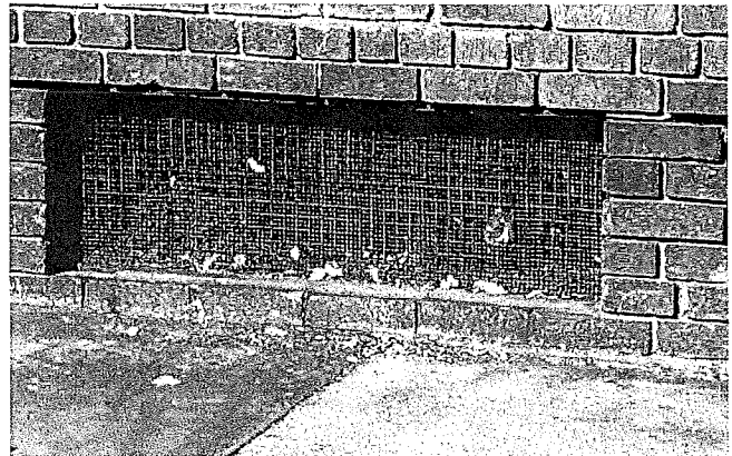
Figure 1. Ventilation grilles; note 1"x1" historic iron grille.
