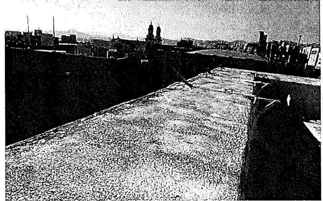
Figure 1. Parapet at southwest corner; note roofing membrane conditions at parapet cap.
