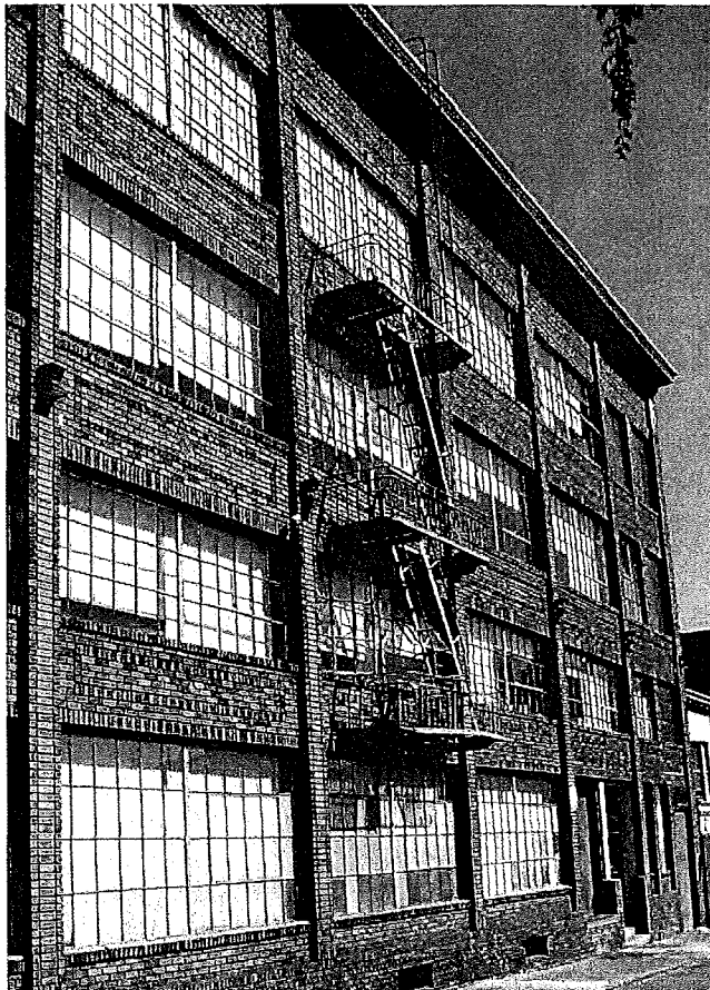
Figure 1. Metal fire escape at south elevation.
