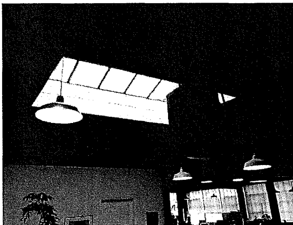
Mezzanine level skylight and exposed ceiling joists. (Page & Turnbull, April 2013)
