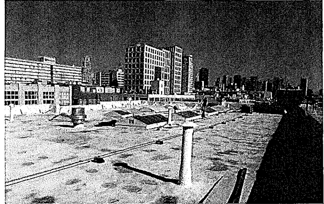
Figure 1. Roof of 149 9th Street, typical.
