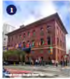
1 University Club 800 Powell Street Year Built: 1908 Significant for its Roman Renaissance Revival architecture designed by San Francisco architects of merit Bliss & Faville originally for Stanford University
