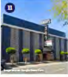
11 Bimbo's 365 Club 1001-1025 Columbus Avenue Year Built: 1981 Significant for its association with Italian American cultural heritage, its Midcentury Modern architecture designed by architect of merit Timothy Pflueger, and as a popular nightclub
