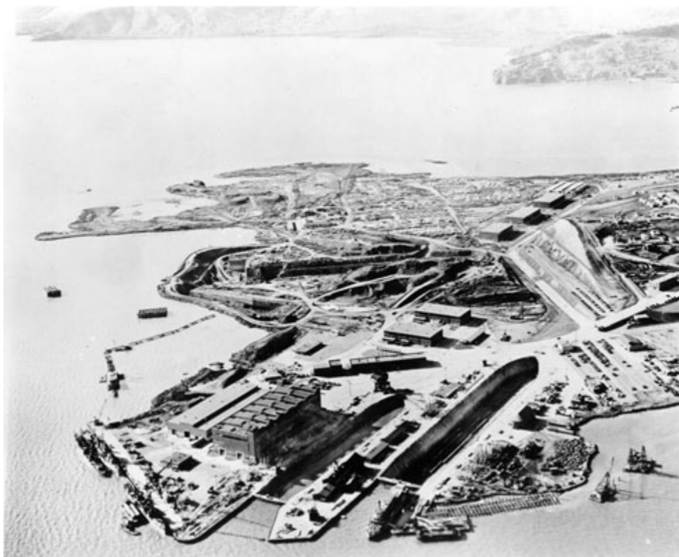
Figure 1: The Shipyard Under Construction
