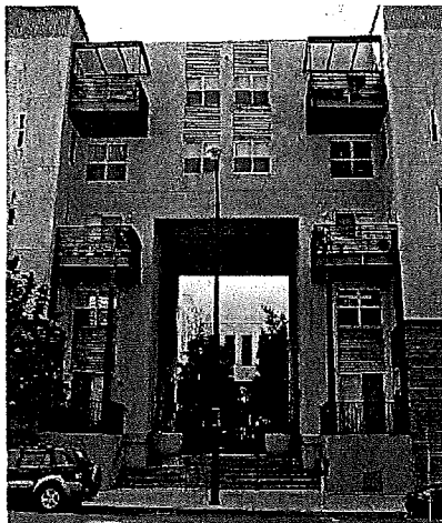
Shared portal entry
