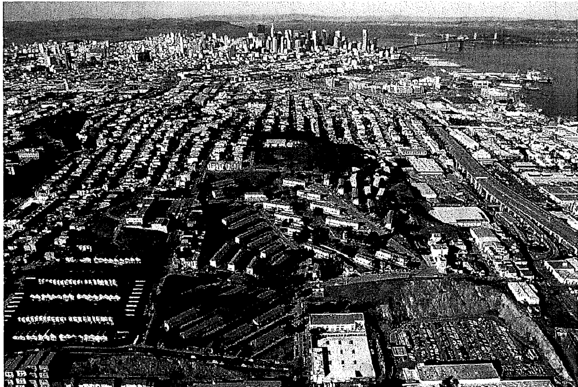
Aerial Perspective: Existing Conditions
