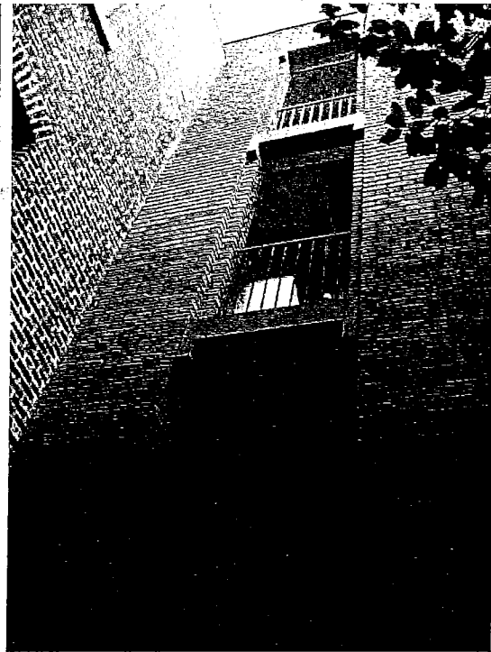
Detail of openings to stairwell on the west façade, looking east. (Page & Turnbull, March 2013)
