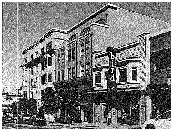
Setting back the upper floor moderates the height and sense of scale between neighboring buildings.
