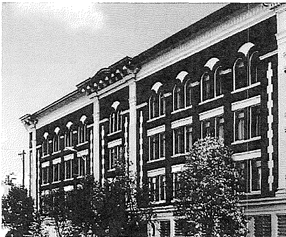
A facade is modulated with the spacing pattern of windows.
