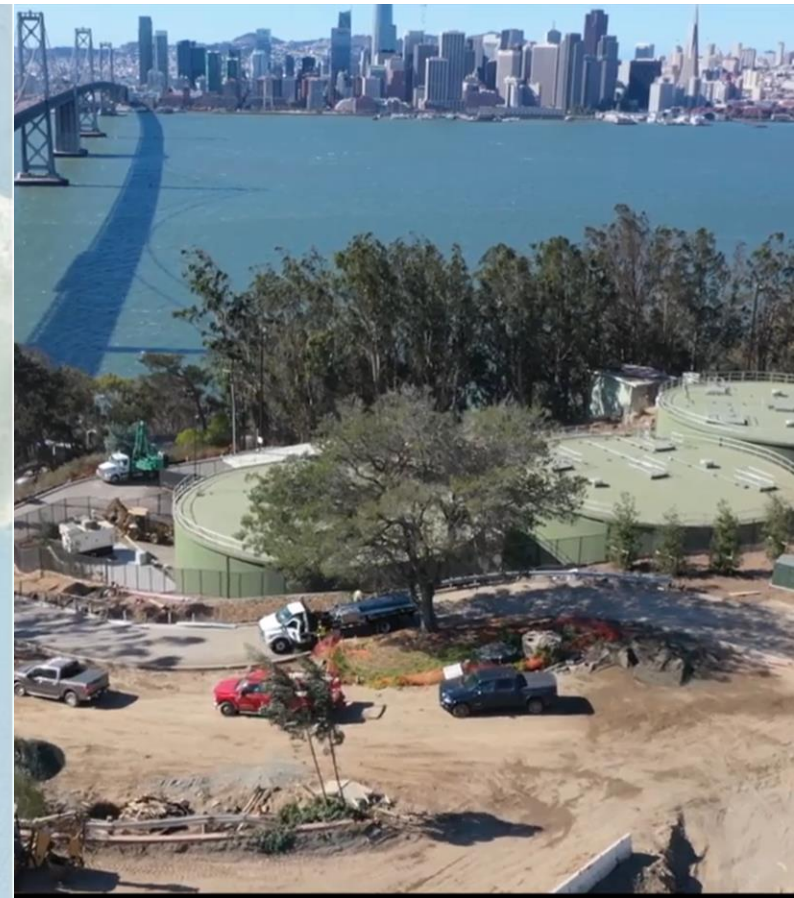
new water tanks
