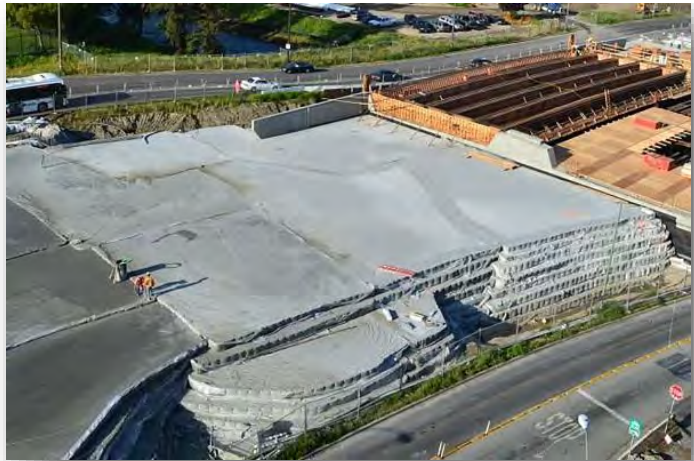
Figure 2. LCC use at Oakland 12th Street Project near Lake Merritt.
