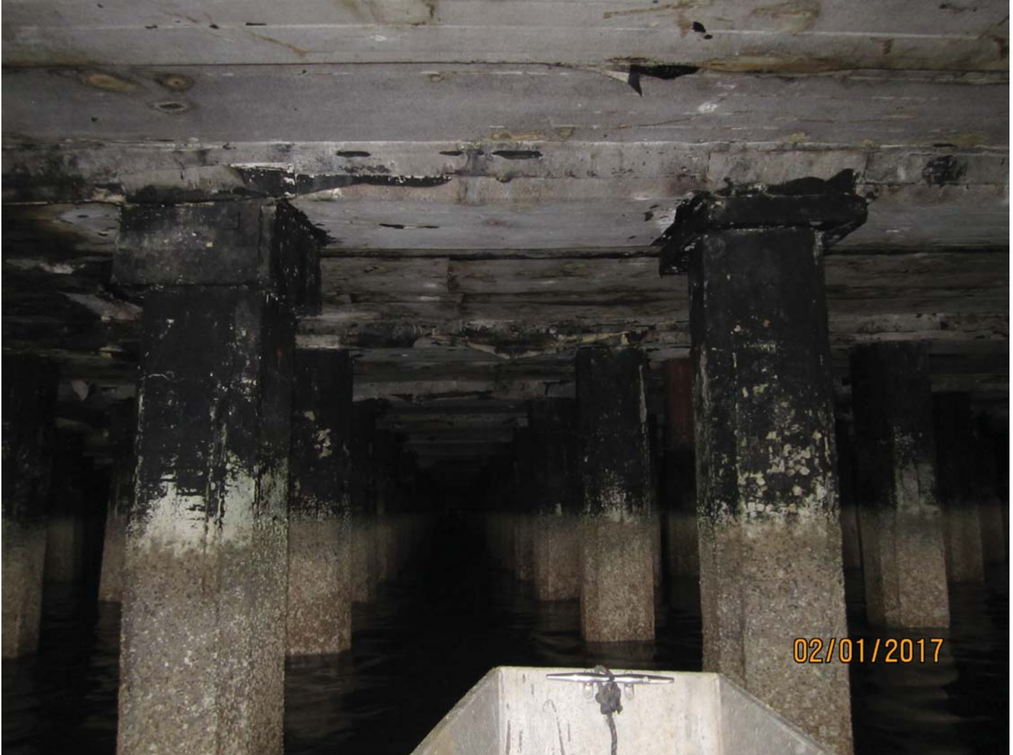
Photo 12. Typical conditions of concrete deck and concrete pile jackets along centerline of pier.
