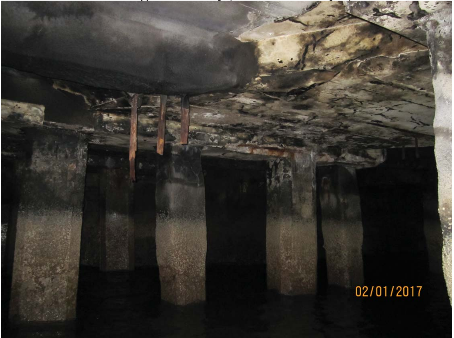
Photo 4. Northern rail track at upper right, concrete surface coated in waterproofing paper.
