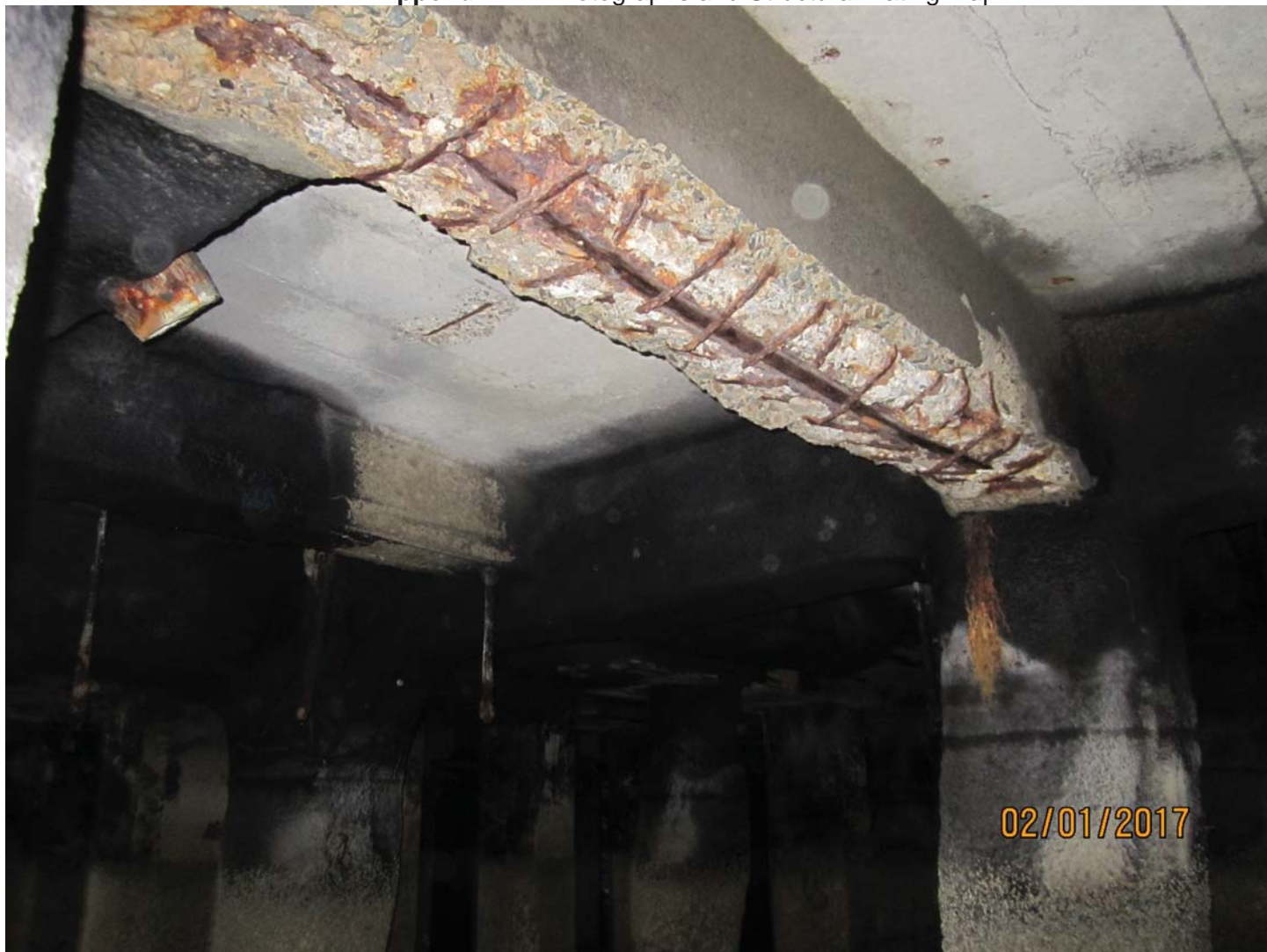
Photo 6. One concrete beam noted with severe spalling. Does not appear to have ever been repaired with shotcrete.
