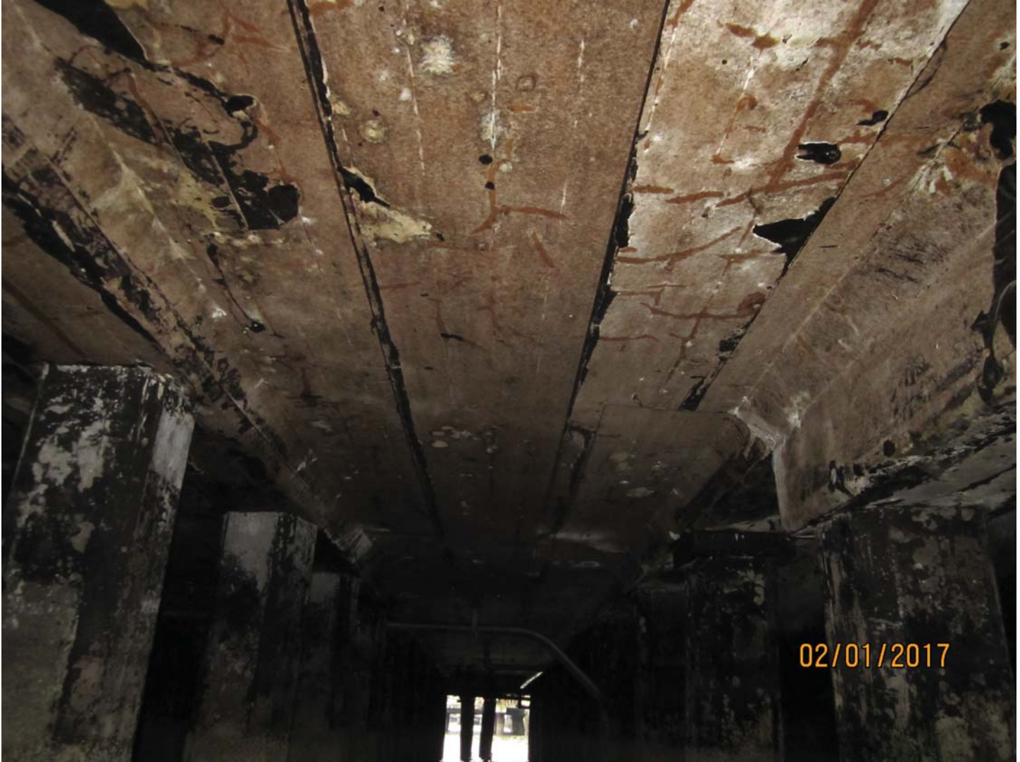
Photo 8. Typical condition of concrete deck. Old waterproofing paper is in varied condition, but appears to have protected the concrete.
