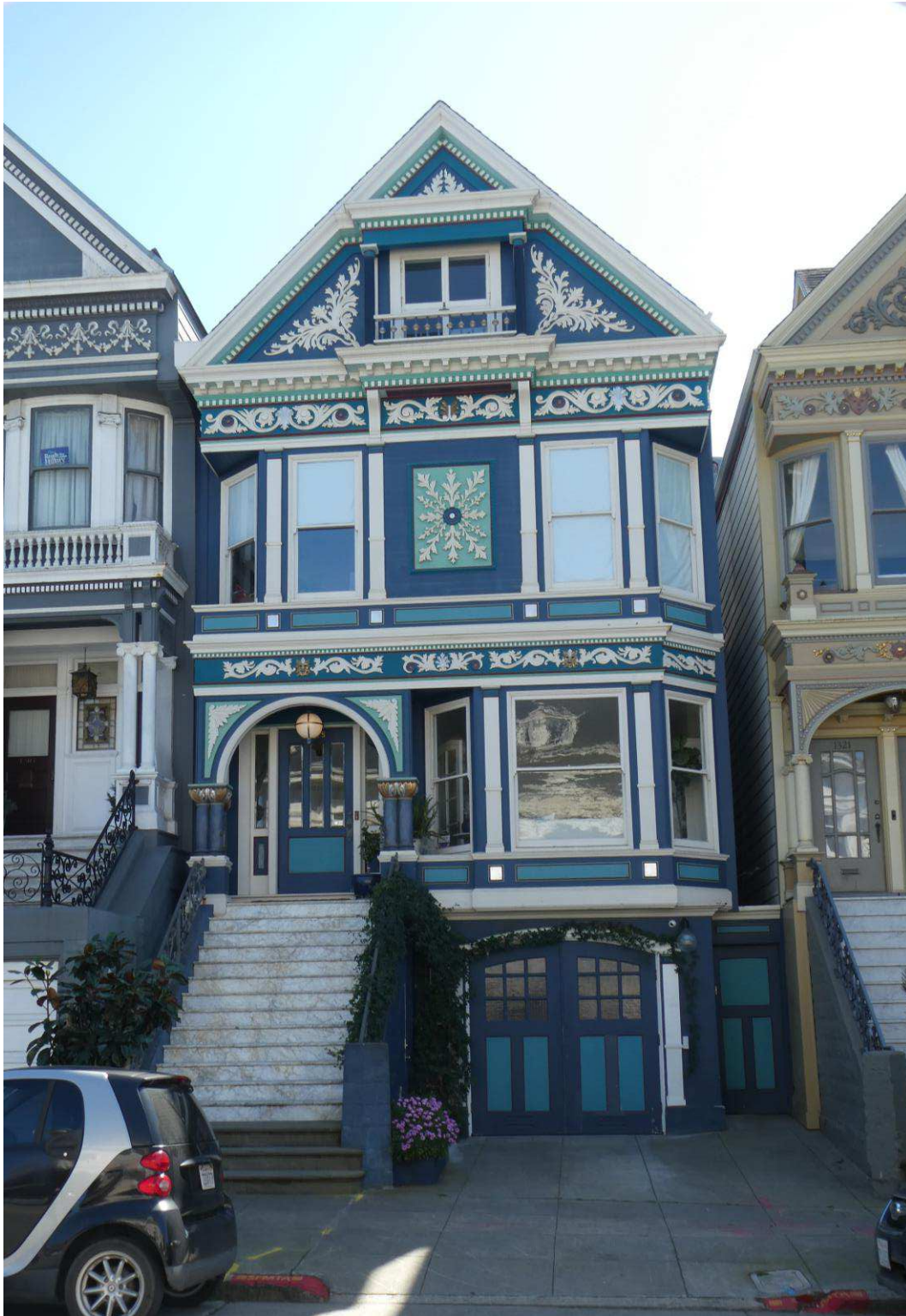
Figure 26. Front northwest façade, view southeast.
