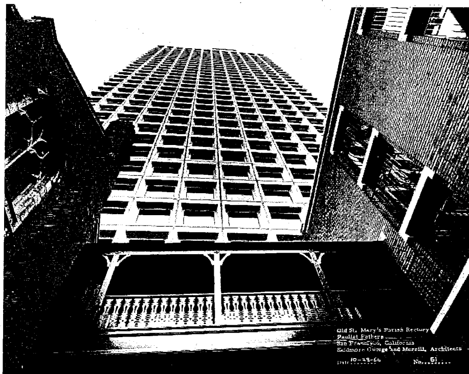
View showing the Sacristy (left), bridge and rectory (right) in relation to the Hartford Building, October 1966. (©Skidmore, Owings & Merrill LLP 2013)
