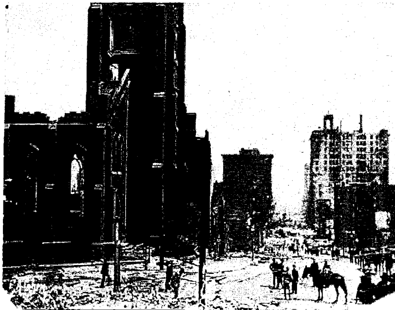
Old St. Mary's following the 1906 Earthquake (SFPL Historic Image AAC-2704)
