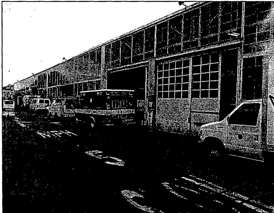
Photograph 7. Building B, camera facing southeast, August 20, 2014.
