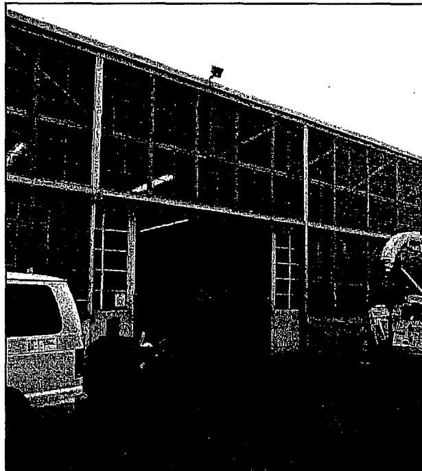
Photograph 5. Building B showing car shop, camera facing northeast, August 20, 2014.
