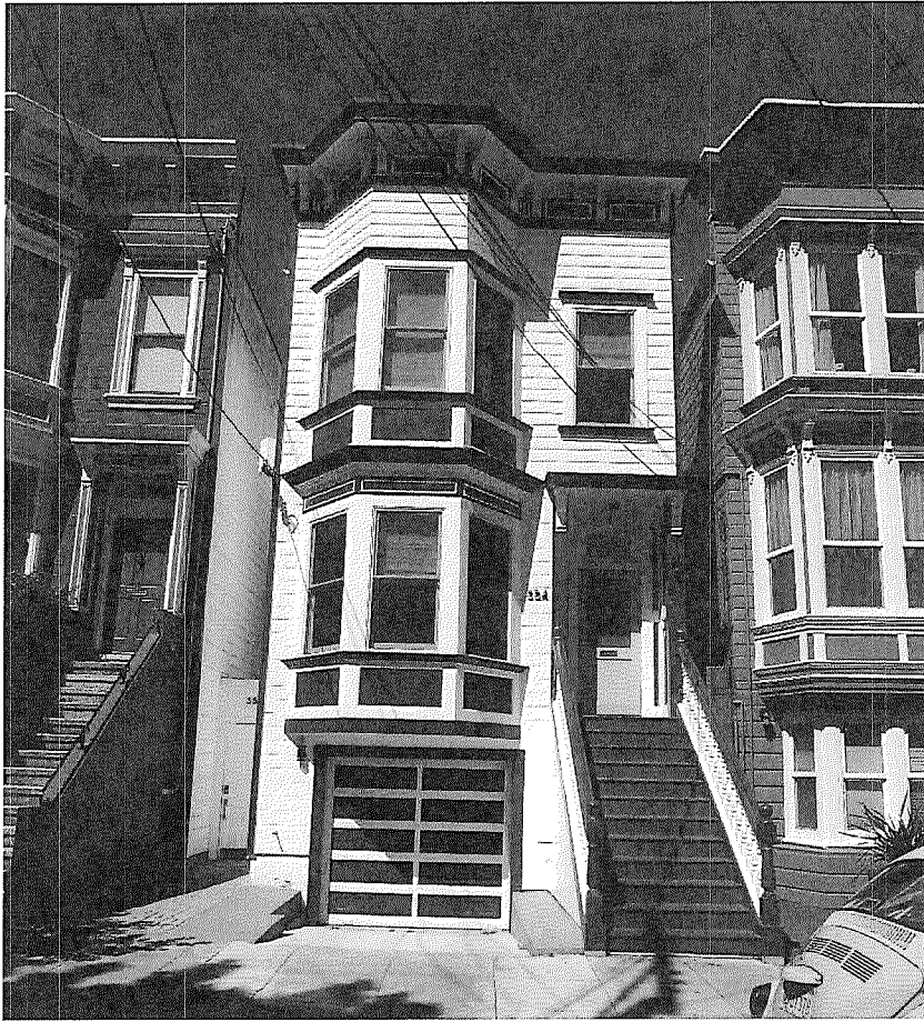
Figure 2. After image of 354-356 San Carlos taken in 2016. Front facade, view looking east.
