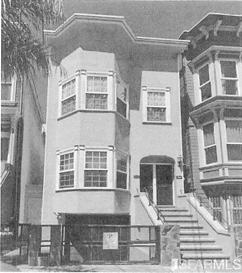
Figure 1. Before image of 354-356 San Carlos St. taken in 2012. Front facade view looking east.
