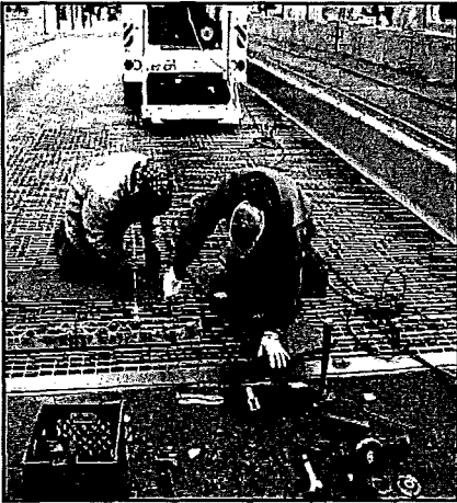
Bridge Deck Repair
