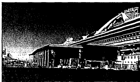
Cruise Terminal at Pier 27
