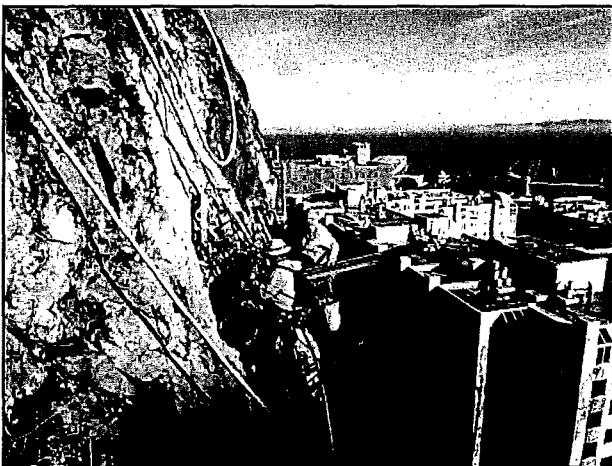
Telegraph Hill rockslide repairs
