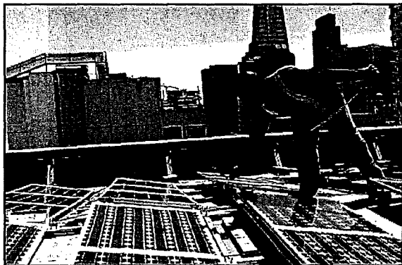
Solar Panel Installation
