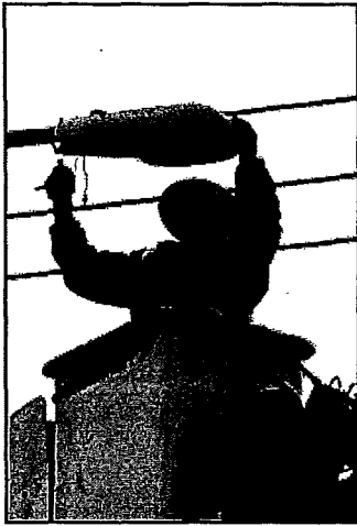
LED Streetlight Installation
