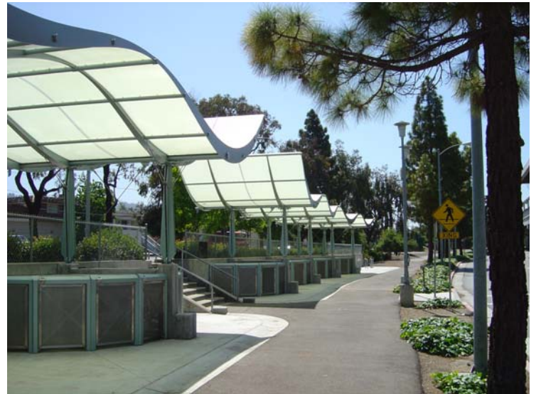
COMMUTER & RECREATIONAL PARKING OHLONE GREENWAY/PLAZA BART STATION EL CERRITO CALIFORNIA
