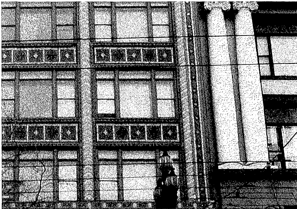
10. April 2017, Exterior Detail, North Elevation, Third Floor, Window at West, Looking S
