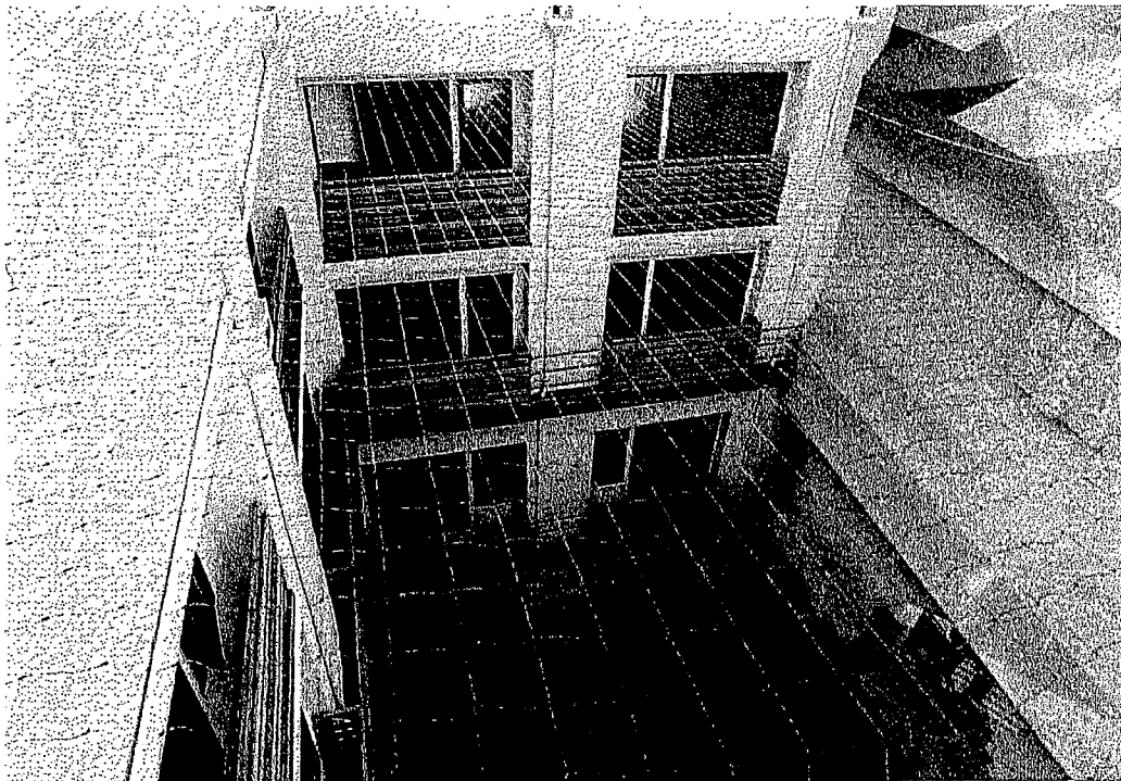
32. April 2017, Lightwell at Center-West, Looking SW
