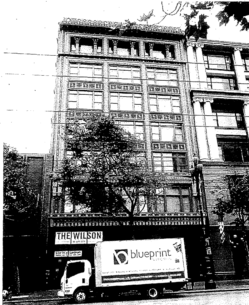
973 Market Street (1900, rebuilt 1906) Sullivan-esque with Byzantine Ornament
