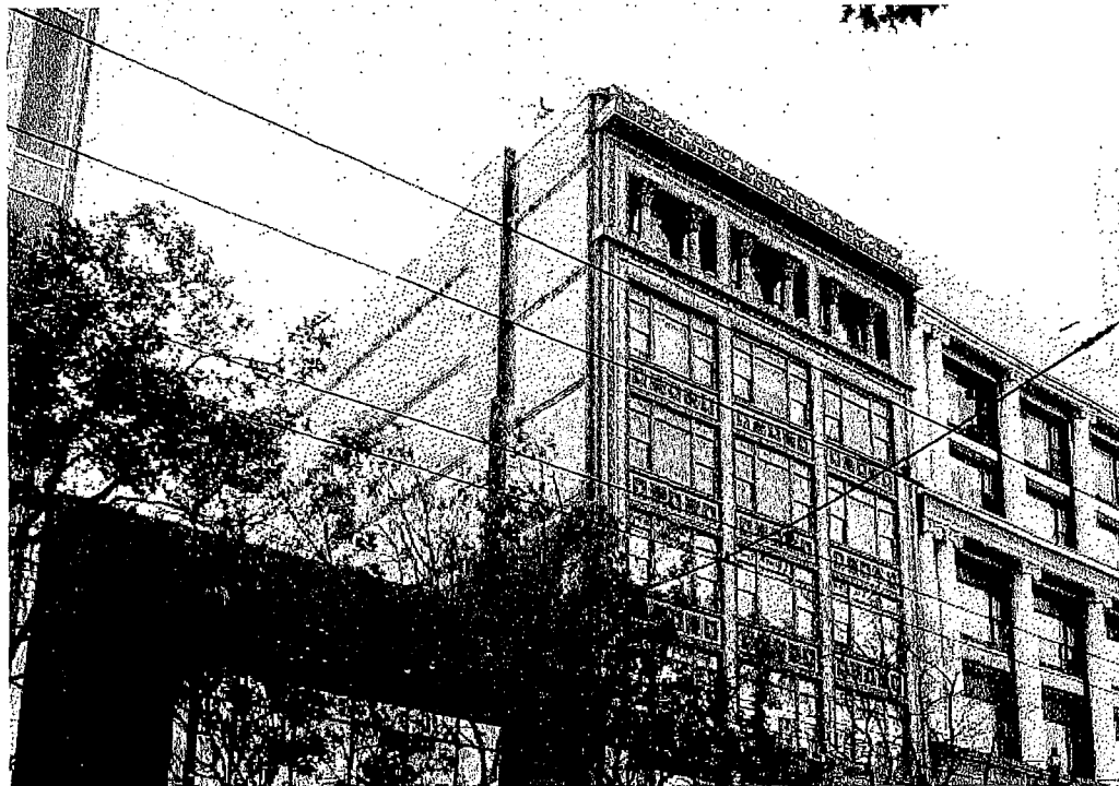
14. April 2017, Exterior View, East Elevation, Looking SW
