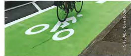
Standard asphalt with green surfacing
