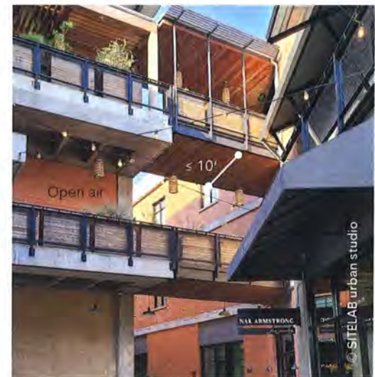
FIGURE 5.38: Pedestrian bridge examples
