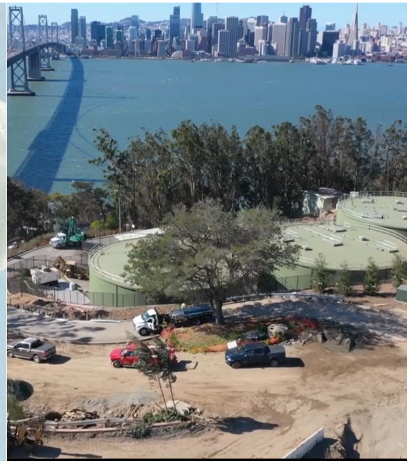
new water tanks
