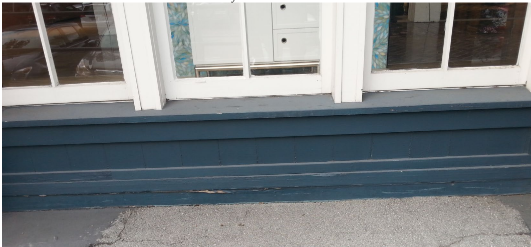
Solid wood bulkhead
