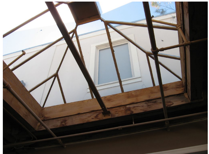
Example of skylight on fourth floor.
