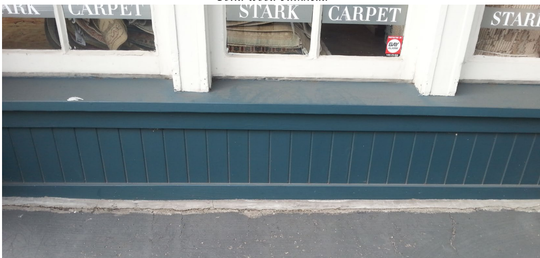
Vertical board bulkhead
