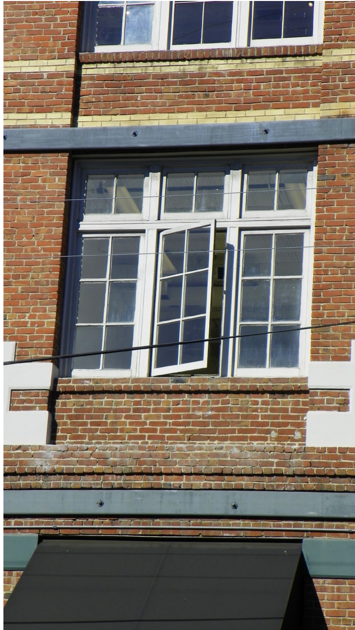
Typical upper story windows
