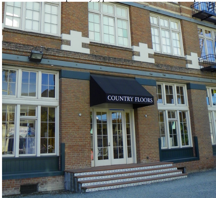
Detail: Contemporary exterior stair, northwest facade
