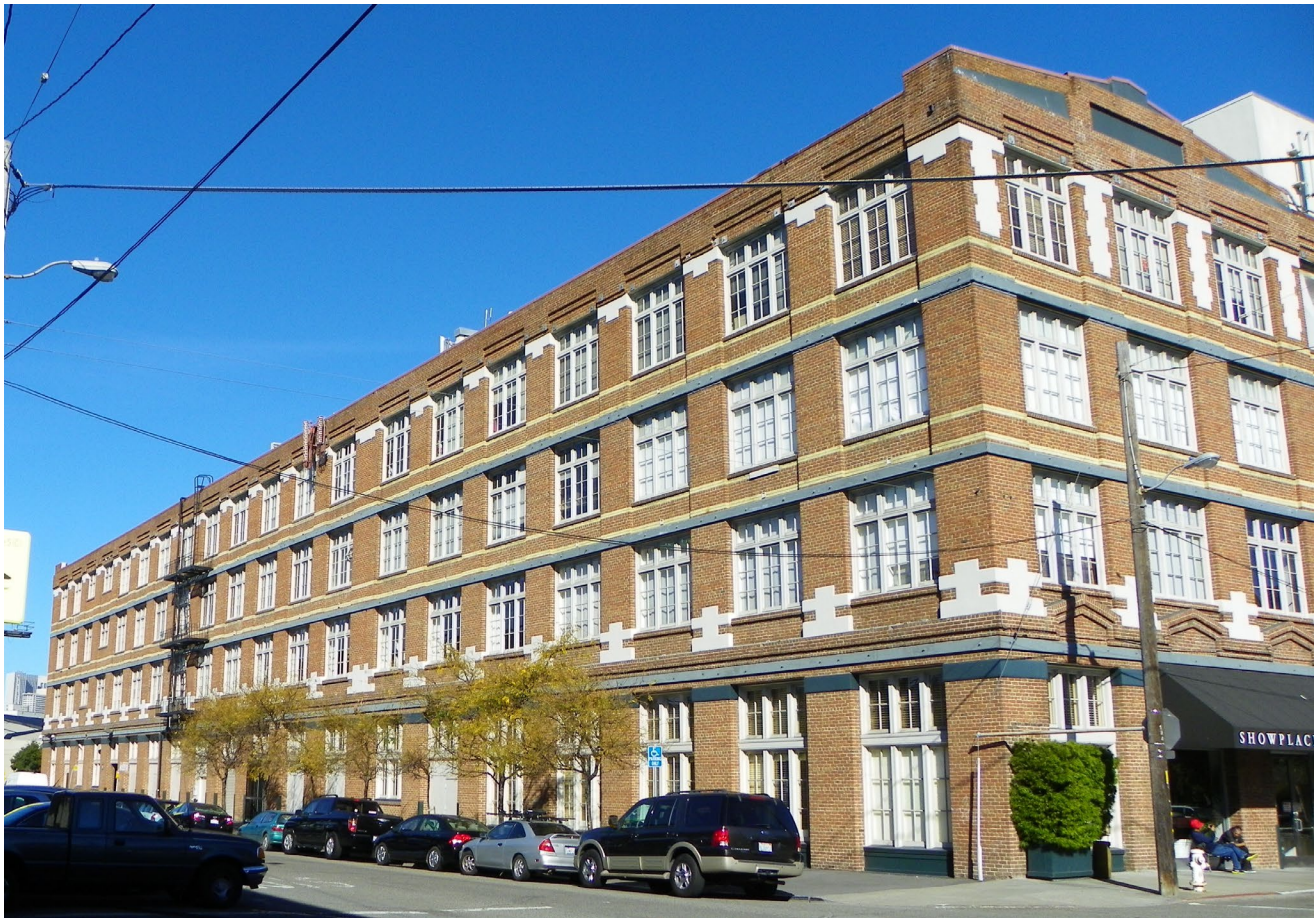
West facade (l), south facade (r)
