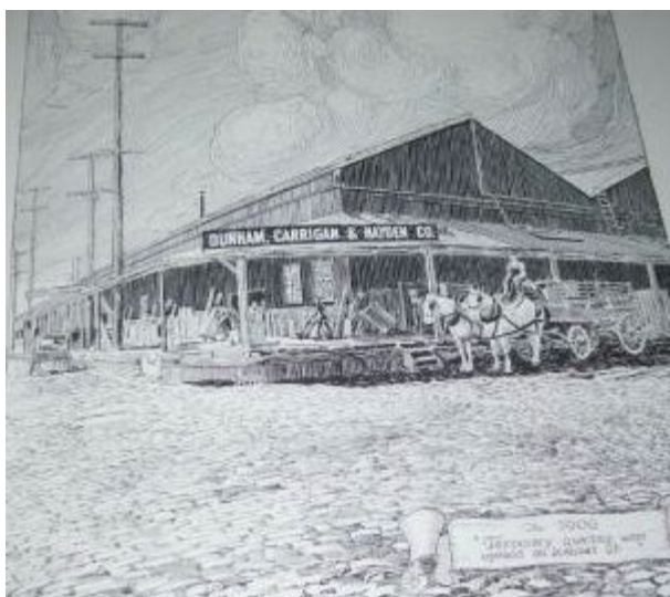
Temporary Dunham, Carrigan & Hayden building view southwest from Alameda and Kansas (Henry Adams) streets
