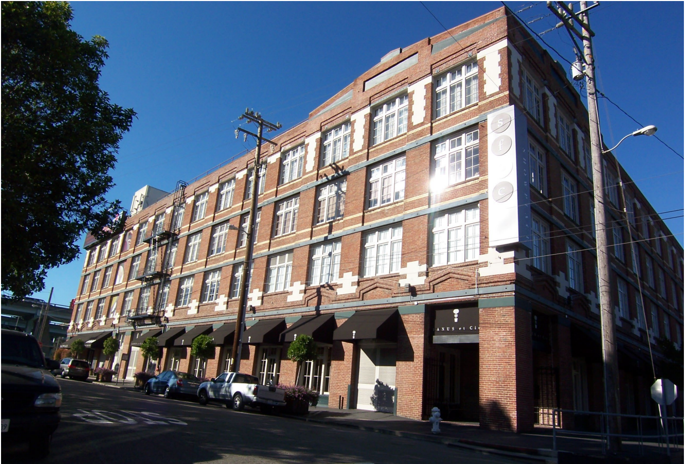
South facade (l), east facade (r)
