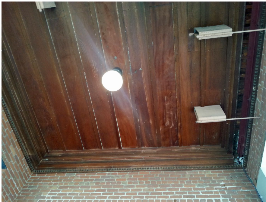
Above: detail, paneled ceiling and crown molding, northeast entrance
