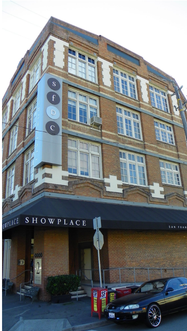
North facade (r) east facade (l)
