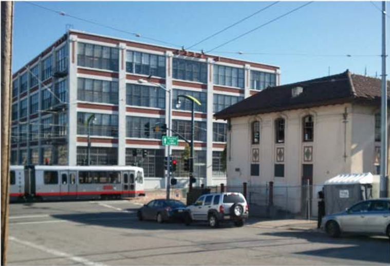
American Can Building with Historic Police Station
