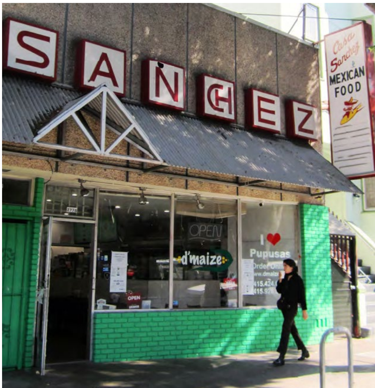
Casa Sanchez, primary façade, view northeast, 2016. Source: Casa Sanchez National Register Nomination
