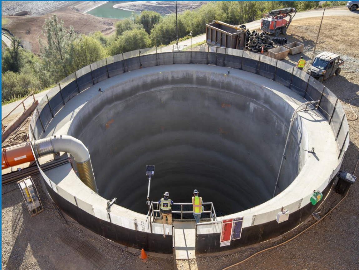
Flow Control Facility Shaft Under Construction
