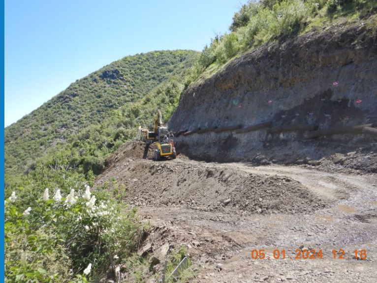
Adit 8/9 Cut Wall
