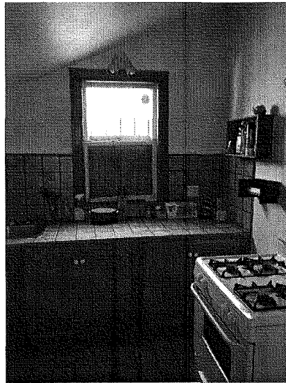
EXISTING BUILDING- KITCHEN
