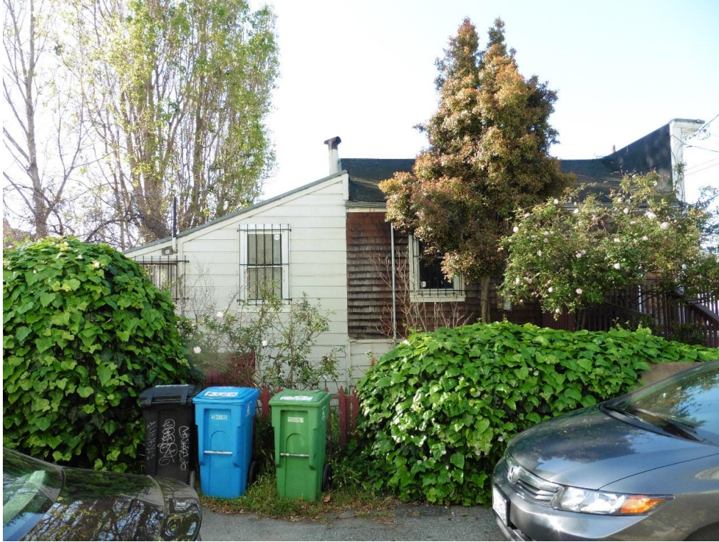
Figure 8. North façade, looking south.
