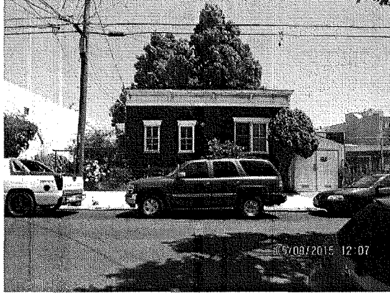
EXISTING BUILDING- LOOKING EAST
