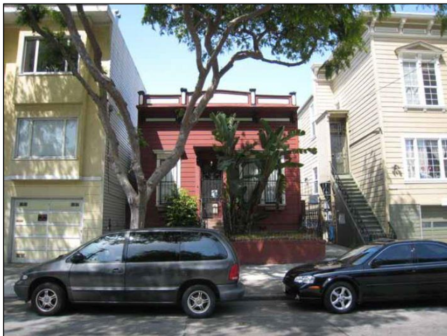
Figure 8 – 2756 Folsom Street – This simple vernacular Italianate cottage was identified as being individually eligible for listing in the California Register. The property retains its original massing, form, and fenestration pattern, and architectural details.
