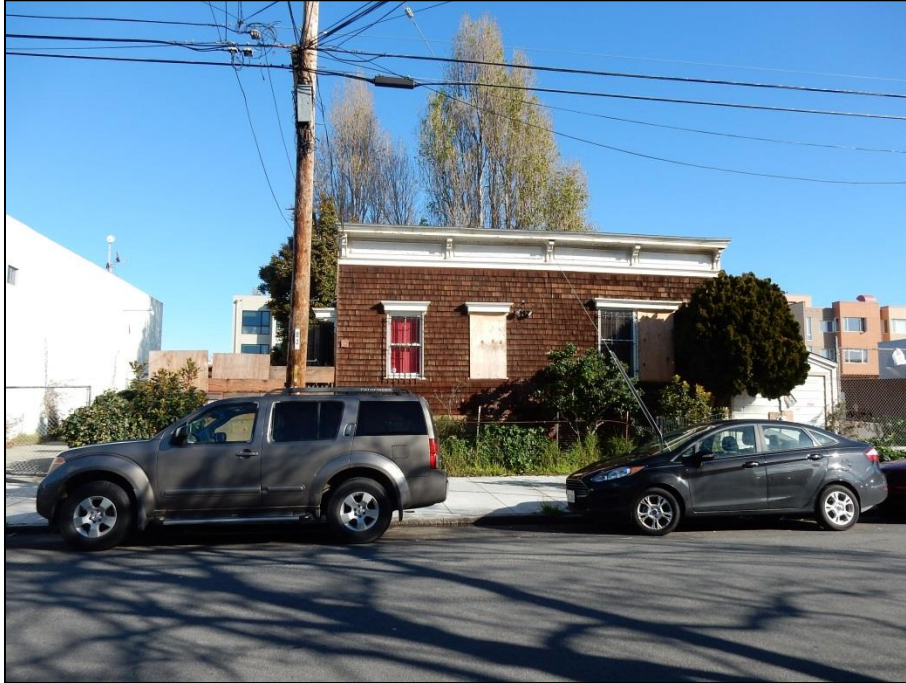
Figure 1 – 953 Treat Ave – Primary façade (west elevation) showing alterations including expansion of the original building to the south which resulted in the irregular fenestration pattern, addition of shingles, and shed addition to the south (left).
