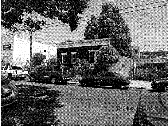
EXISTING BUILDING- LOOKING NORTHEAST
