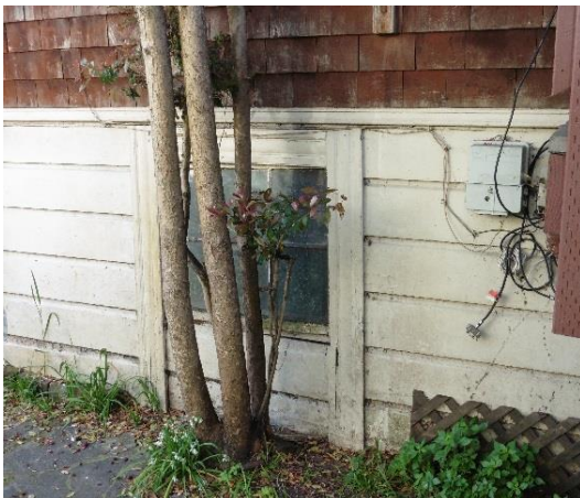
Figure 9. Window to crawlspace at north façade.
