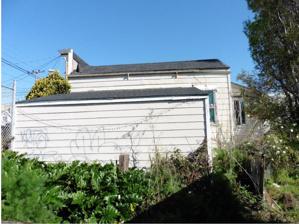
Figure 21. South façade, looking north.
