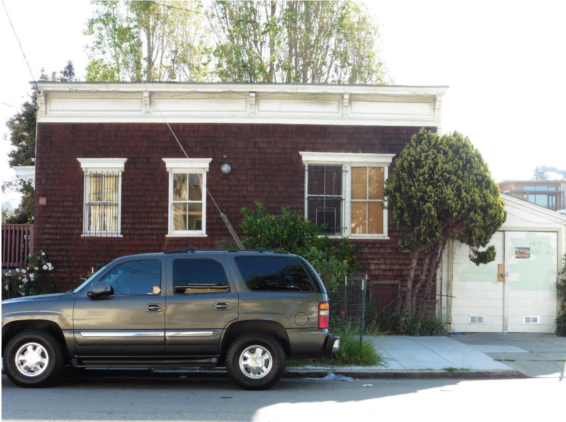
Figure 4. Primary false front façade, looking east.
