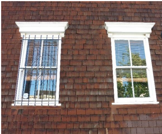
Figure 5. Primary façade windows.
