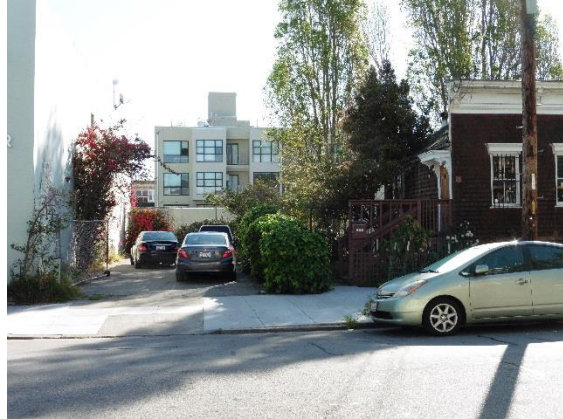
Figure 24. Paved northern portion of subject lot, looking east.
