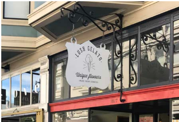
Signage has the ability to enhance the architectural character of the building.
