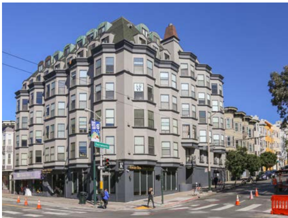
Sloping the roof helps the massing of this building transition to the scale of the adjacent lower buildings.
