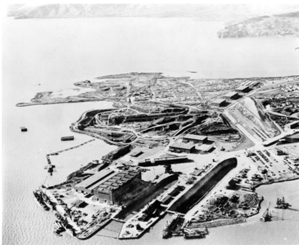
Figure 1: The Shipyard Under Construction
