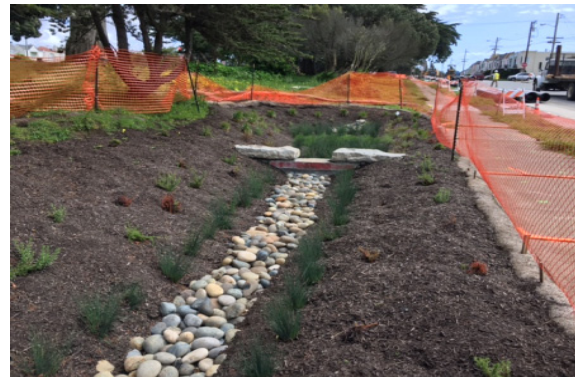
Sunset Phase 1 rain garden located along Sunset Blvd. between Vicente and Wawona streets
