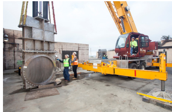
WW-572R - new hydraulic operated 54-inch Knife Gate Valve installation
