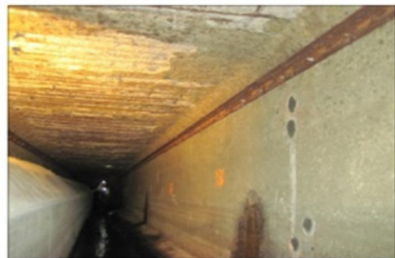
Interior of Jackson Street Box Sewer
