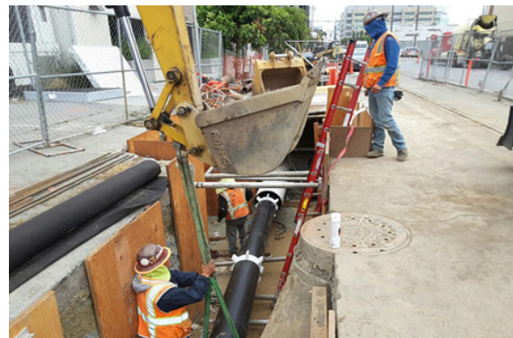
Insertion of the HDPE Force Main
