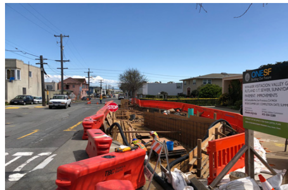
Rain Gardens being constructed at Sunnydale Avenue and Rutland Street
