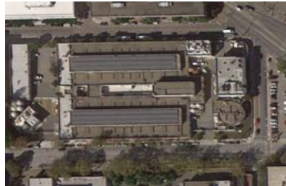
Existing North Point Facility Pump Station
