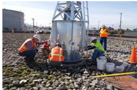
At the Existing Wastewater Treatment Plant, installation of a new rock trickle filter rotary distributor arm was completed in the Summer of 2016.
