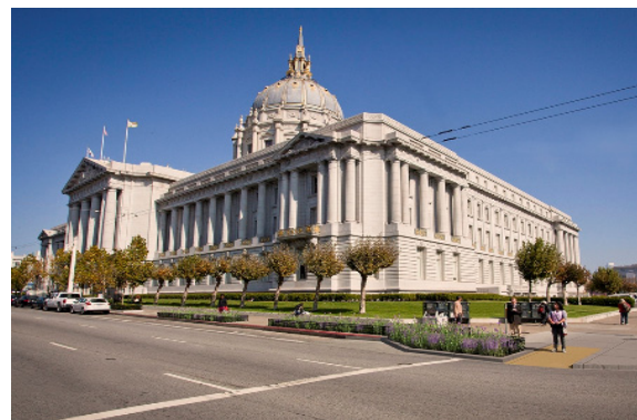
Van Ness BRT – Rendering of proposed green infrastructure rain gardens along City Hall
