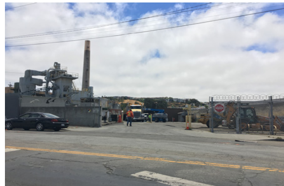
Asphalt plant after salvage
