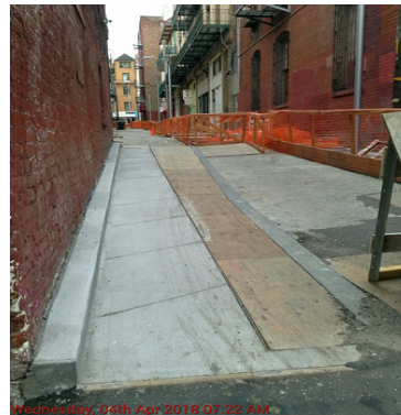
Spofford Alley, pouring regraded road base
