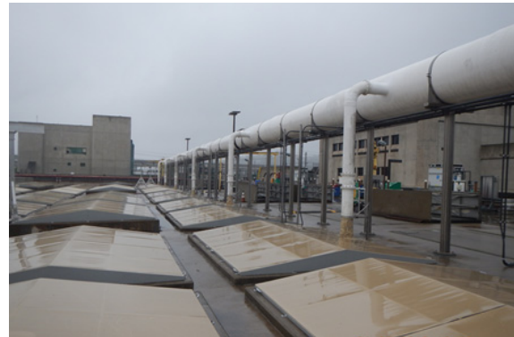
New Primary Sedimentation Tank Odor Control Covers and Ductwork
