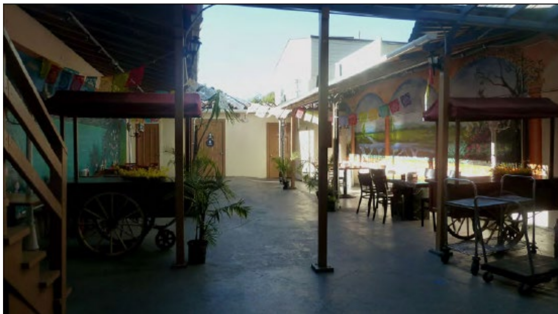
Casa Sanchez (2778 24 th Street), rear courtyard, view north, 2016. Source: Casa Sanchez National Register Nomination
