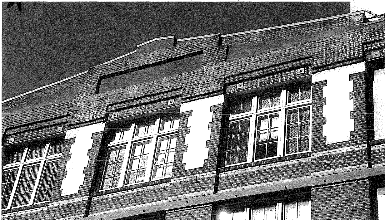
Detail: Peaked parapet and quoin-like panels (south facade)
