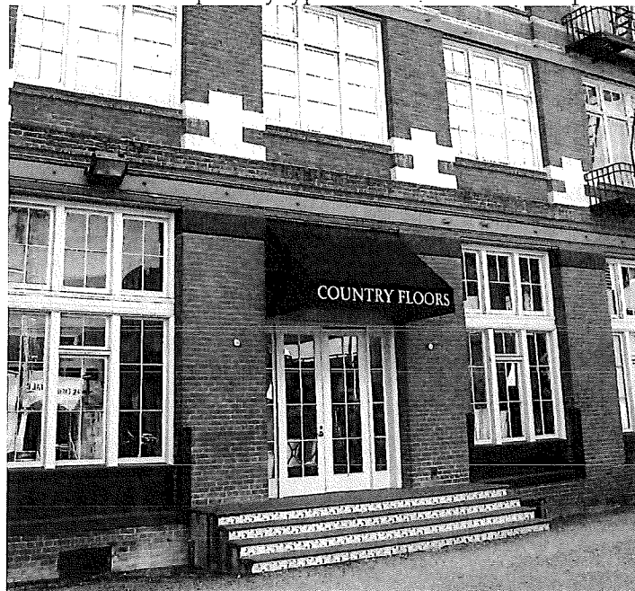
Detail: Contemporary exterior stair, northwest facade
