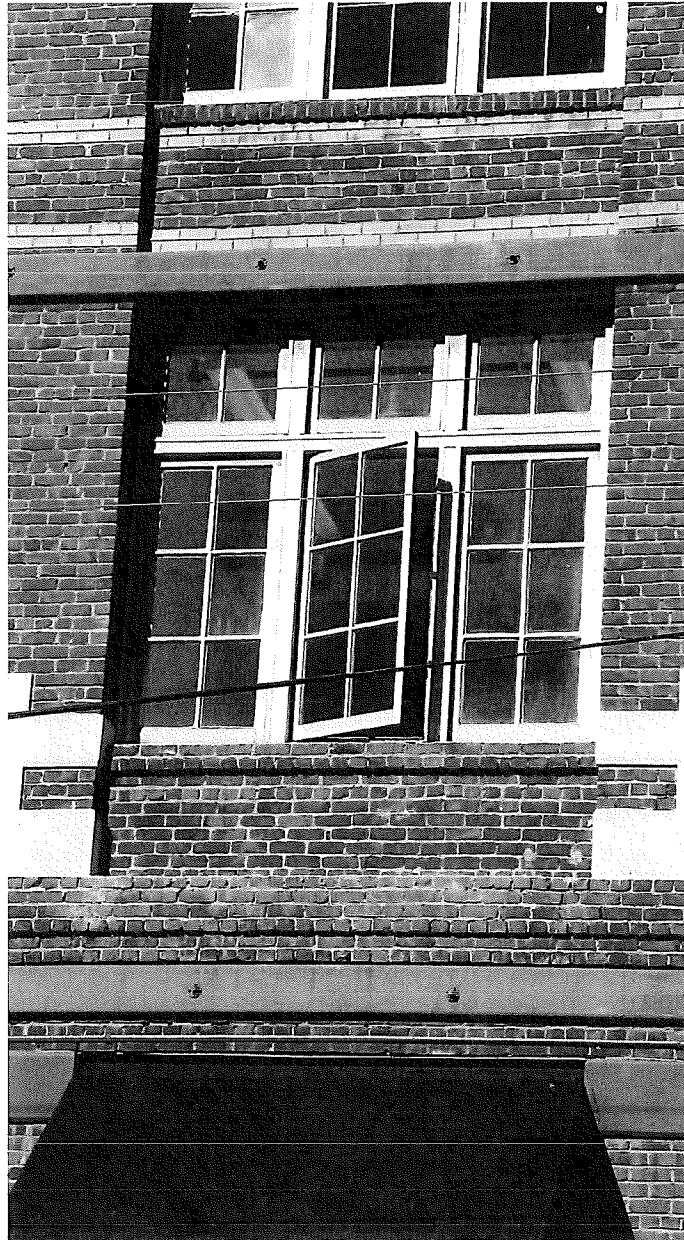
Typical upper story windows
