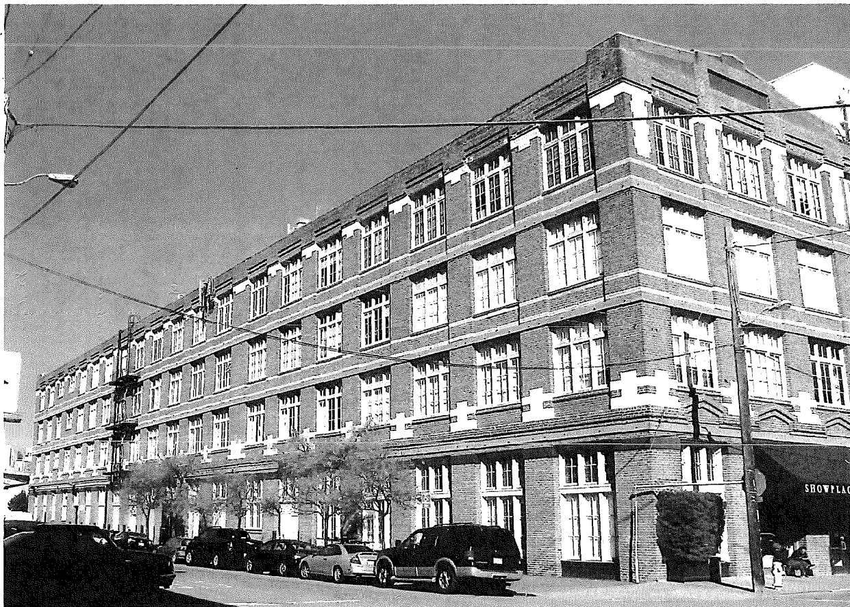
West facade (l), south facade (r)
