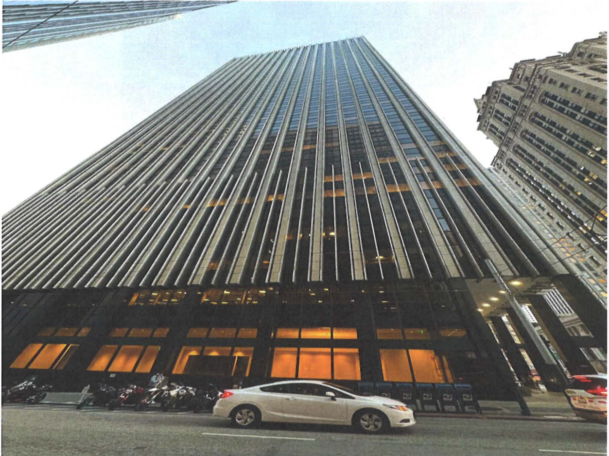
Subject block of Market Street showing 44 Montgomery Street (December 2024)
