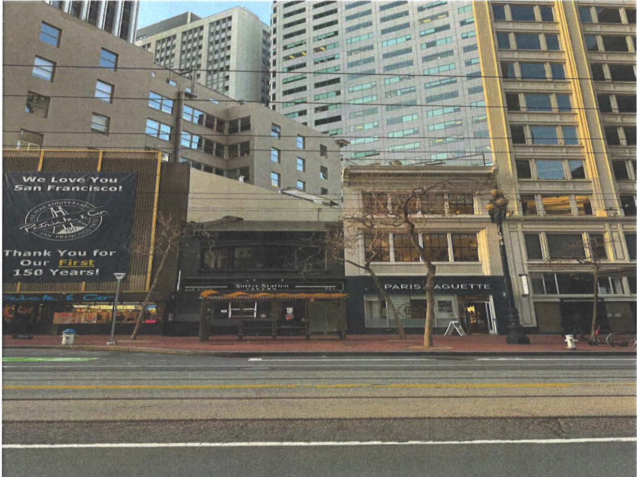
Subject block of Market Street (December 2024)
