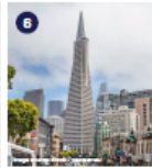
Transamerica Pyramid 600 Montgomery Street Year Built: 1976 Significant for its Brutalist architecture designed by architect of merit William Pereira & Associates
