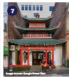
Chinese Telephone Exchange 748 Washington Street Year Built: 1909 Significant for its association with Chinese cultural heritage as the only Chinese telephone exchange in the United States
