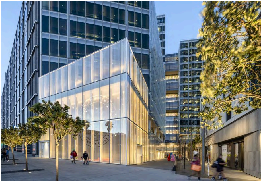
Figure 8: Permit Center at 49 South Van Ness
