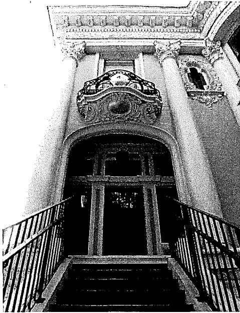
Figure 14: Molded balcony with flanking engaged columns.
