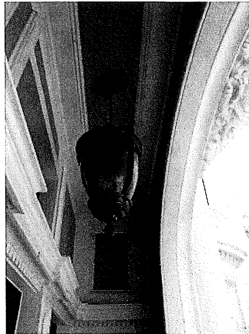
Figure 10: Recessed entry area to Units 2731 and 2733.
