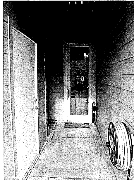
Figure 28: Storage door and south façade access door. door.
