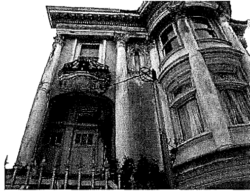
Figure 53: Page & Turnbull 2008 DPR 523A form. Source: South Mission Historic Resource Survey.
