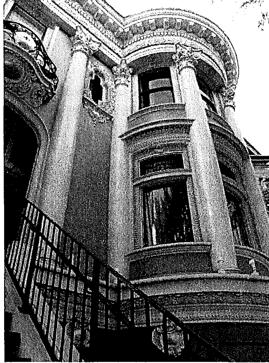
Detail of primary (west) façade
