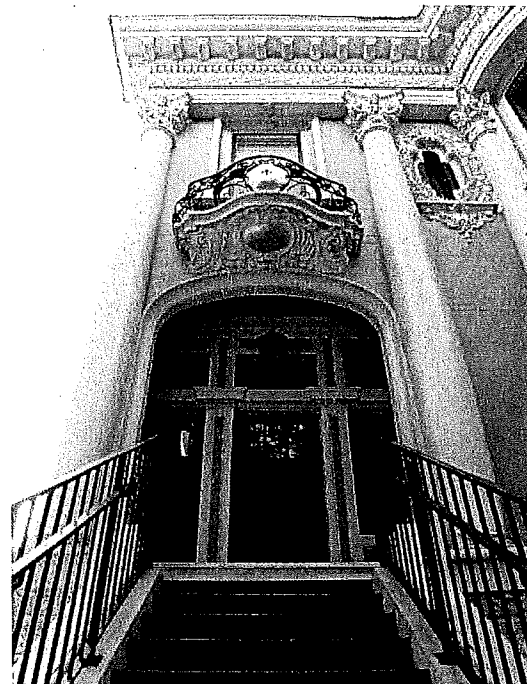
Detail of entry to upper floors
