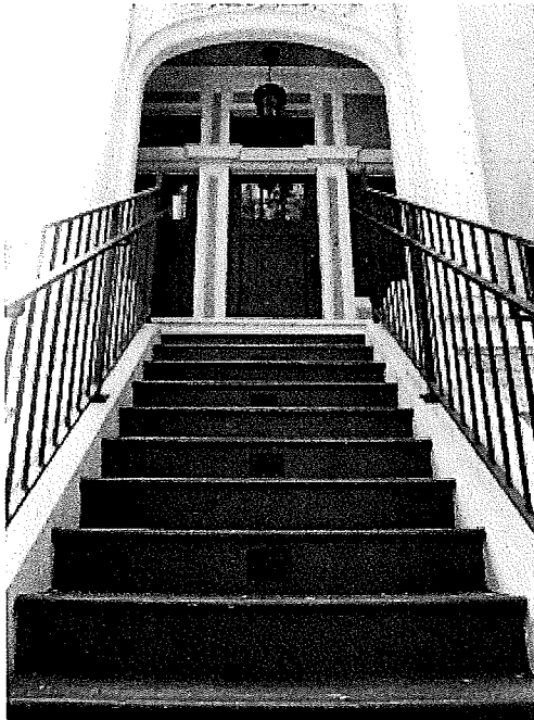
Figure 9: Exterior stairs leading to second story.
