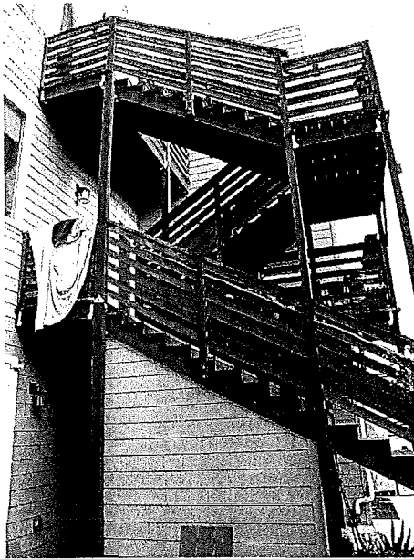
Figure 27: Exterior three-story stairs.
