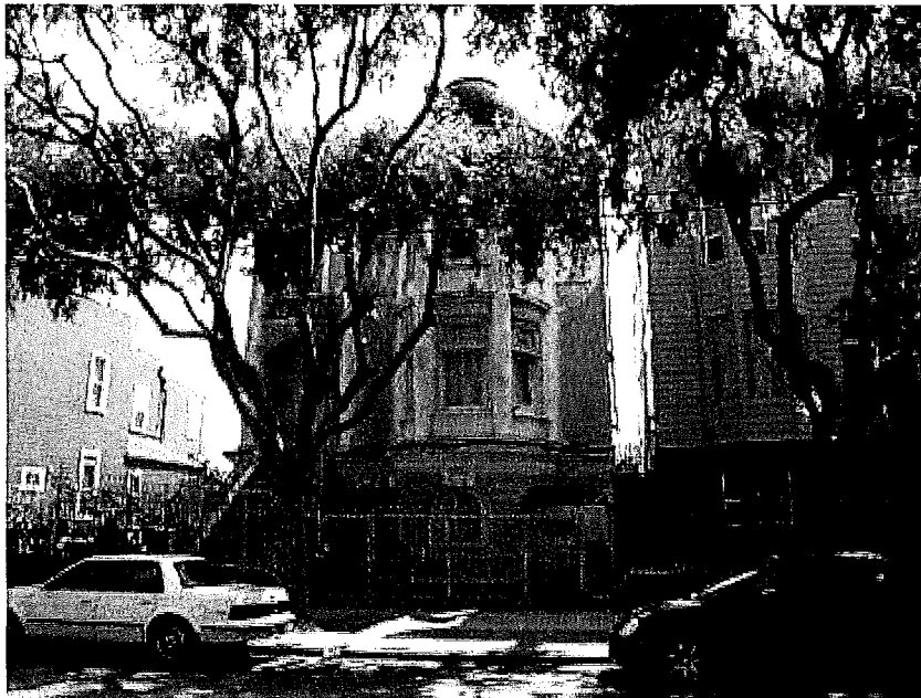
Figure 51: Page & Turnbull 2008 DPR 523A form. Source: South Mission Historic Resource Survey.
