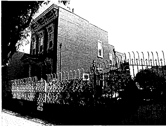
Figure 36: 2721 Folsom Street, looking northeast. Source: Page & Turnbull DPR Form, 2008.
