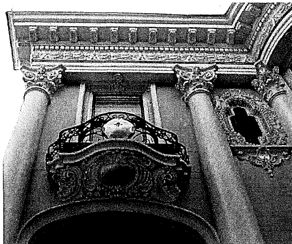
Figure 16: North side of primary façade.
