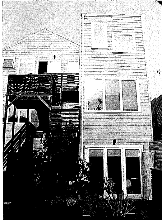
Figure 32: North side fenestration.
