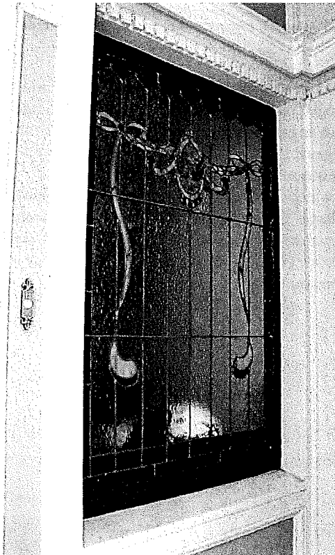
Figure 11: Fixed leaded stained glass window within entry area.
