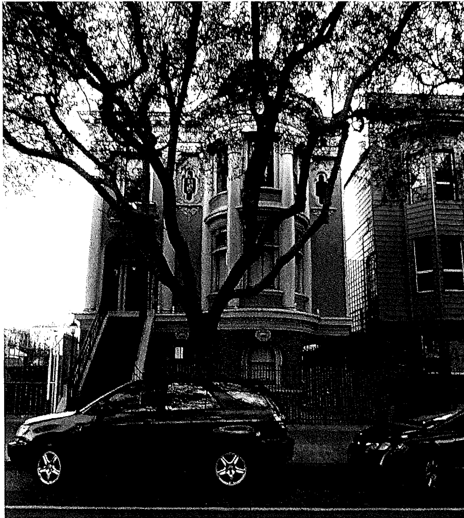
Figure 3: Primary (west) façade of 2731-35 Folsom Street.
