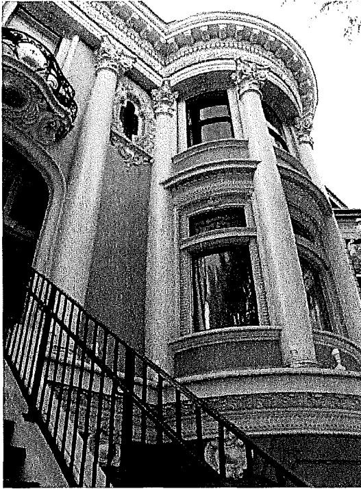
Figure 12: Double height Corinthian engaged columns.
