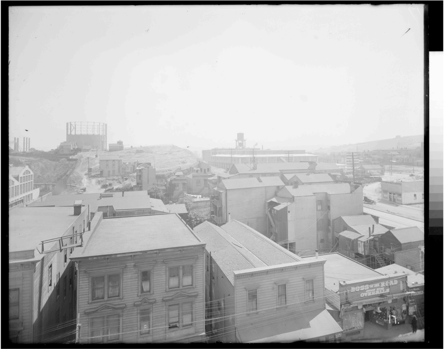
View of Irish Hill property, May 20, 1918. Plate 17. San Francisco Maritime National Historical Park, Bethlehem Steel Corporation, Shipbuilding Division, San Francisco, Calif. photographs, P83-142a.4,574gl (SAFR 17202).
