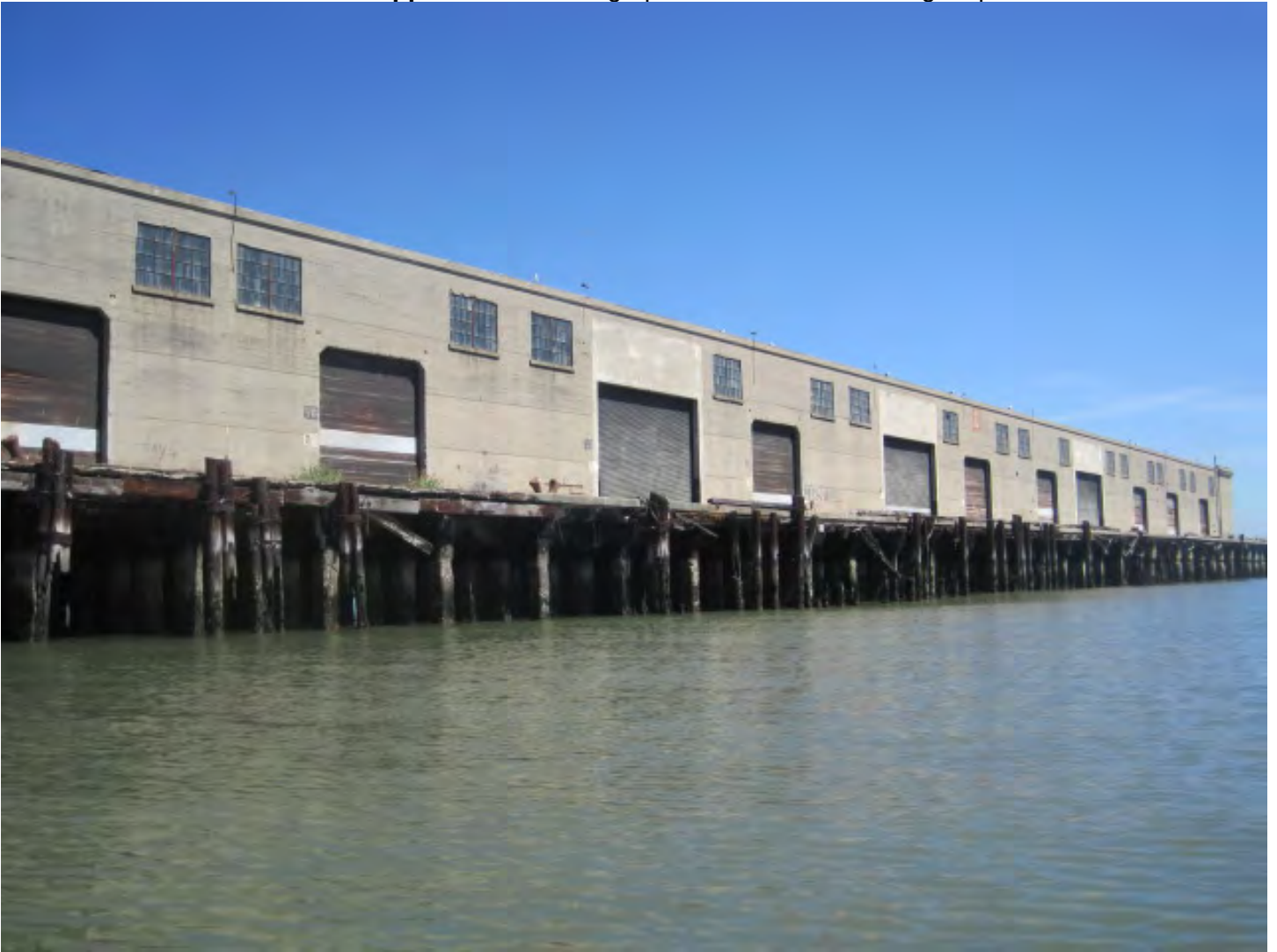
Photo 8. Overall view looking at south side
