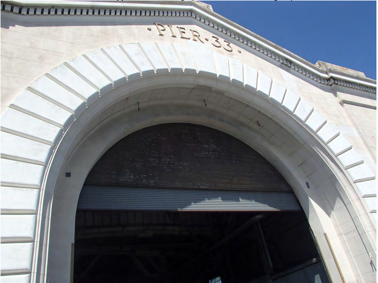
Photo 11. View of south elevation
