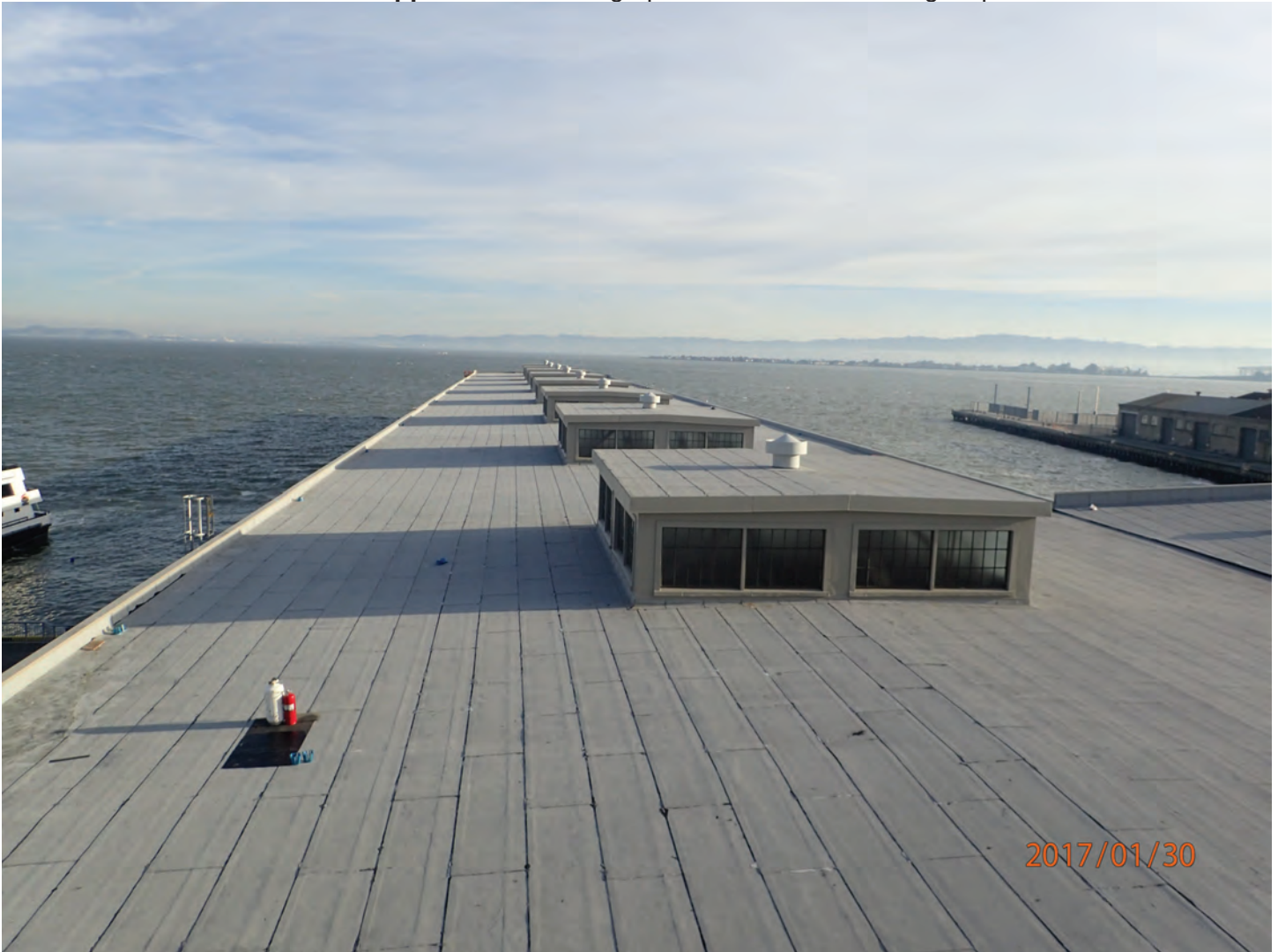
Photo 17. Construction photo of new roofing at Pier 31 shed building.
