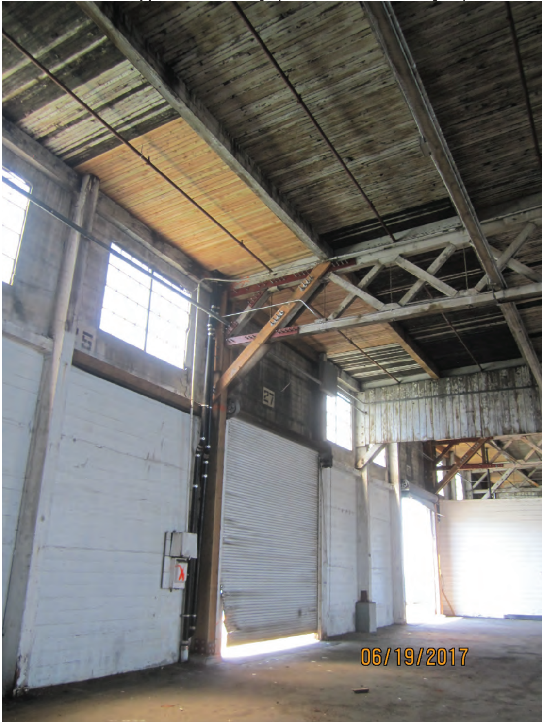
Photo 8. Replacement truss column and strengthened truss connections installed in 2017
