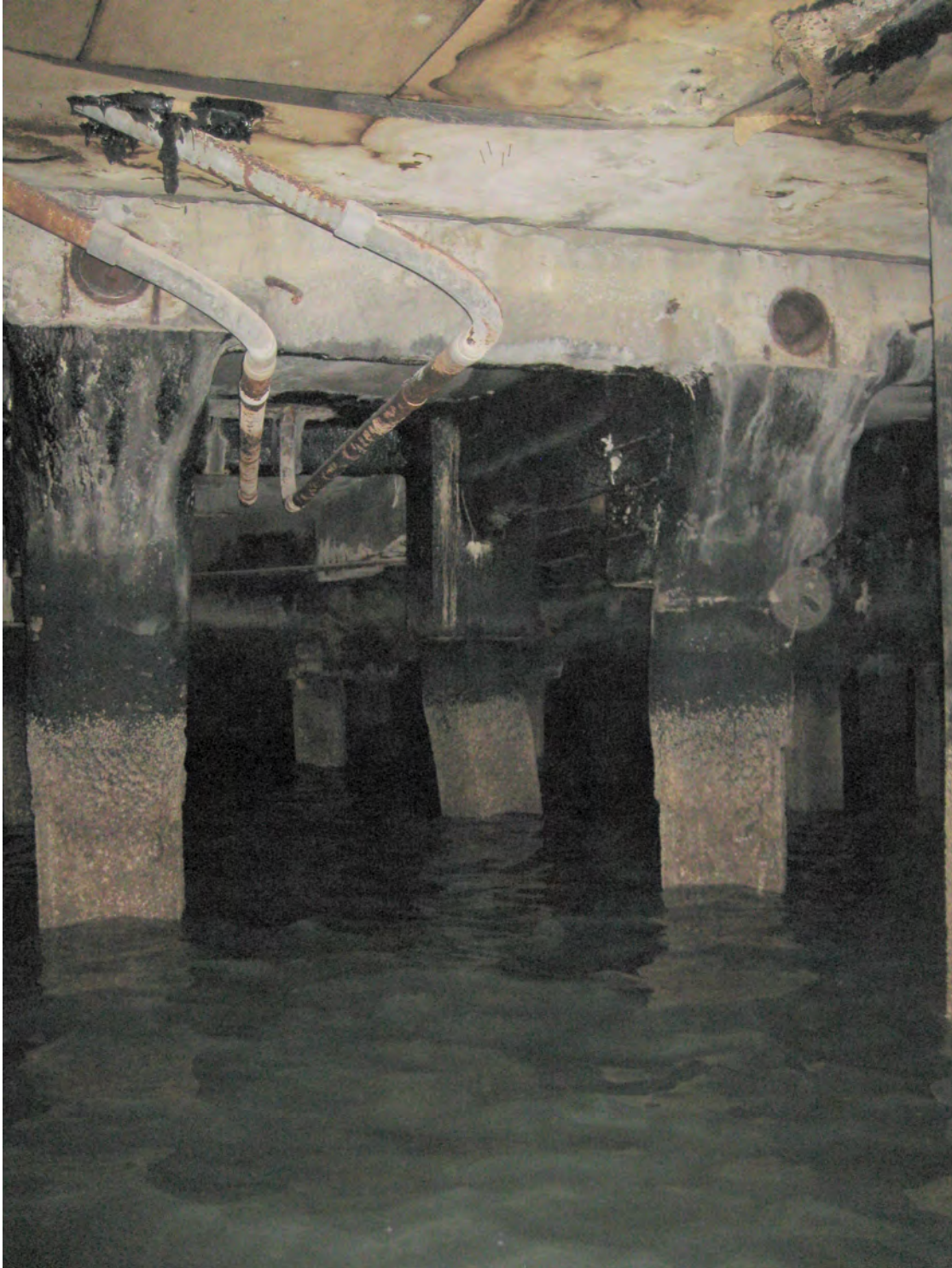
Photo 2. Piles out-of-plumb
