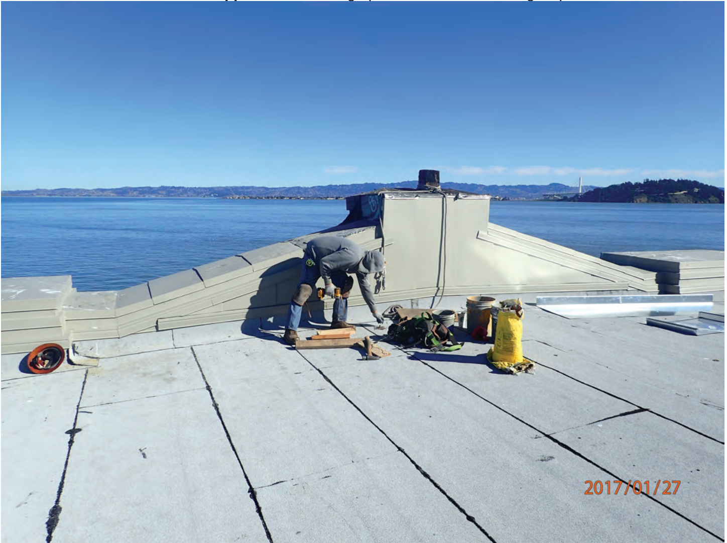
Photo 19. Construction photo of roof work near end of pier.
