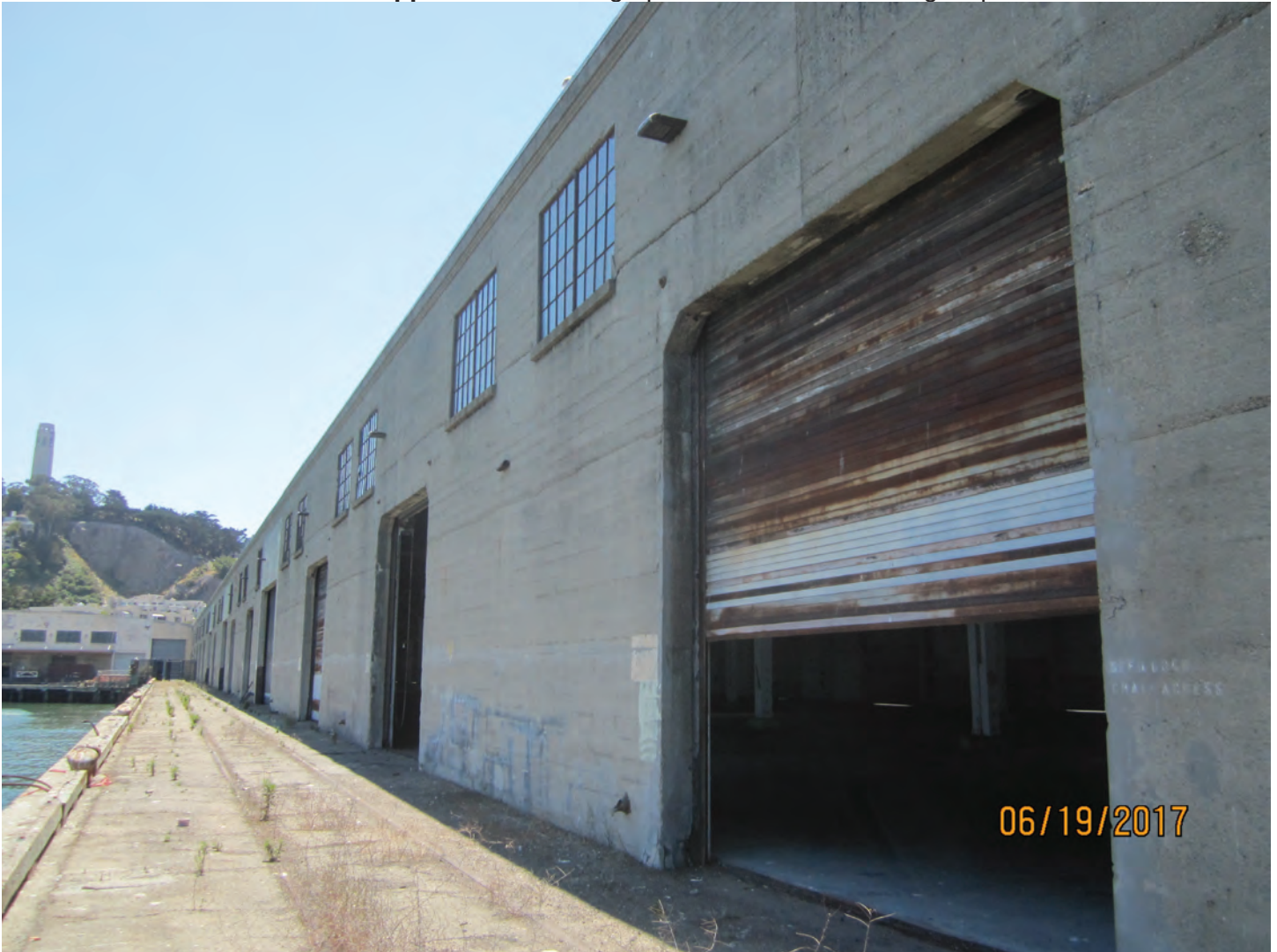
Photo 2. Exterior concrete wall along south face of building.
