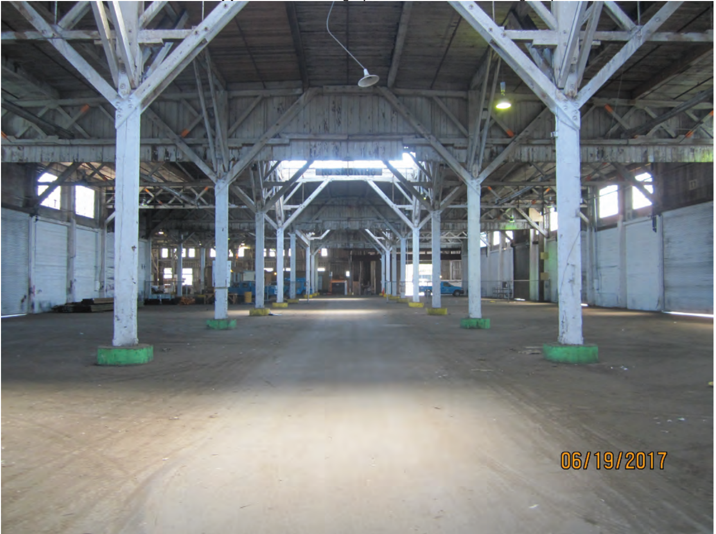
Photo 6. Overall view of shed framing looking towards the Embarcadero
