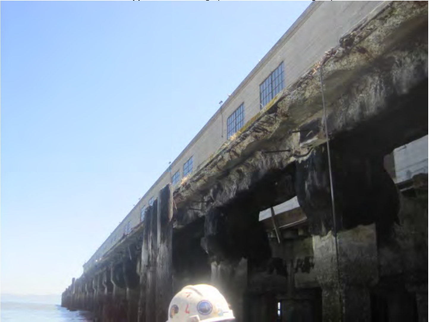
Photo 8. Overall view looking south
