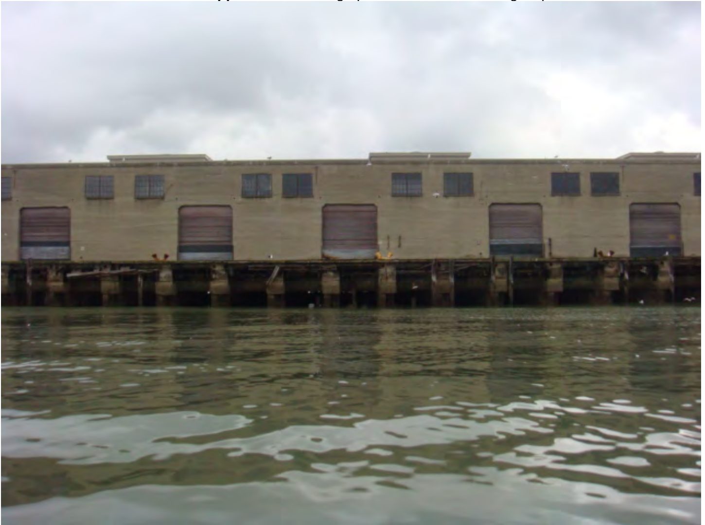
Photo 2. North apron view
