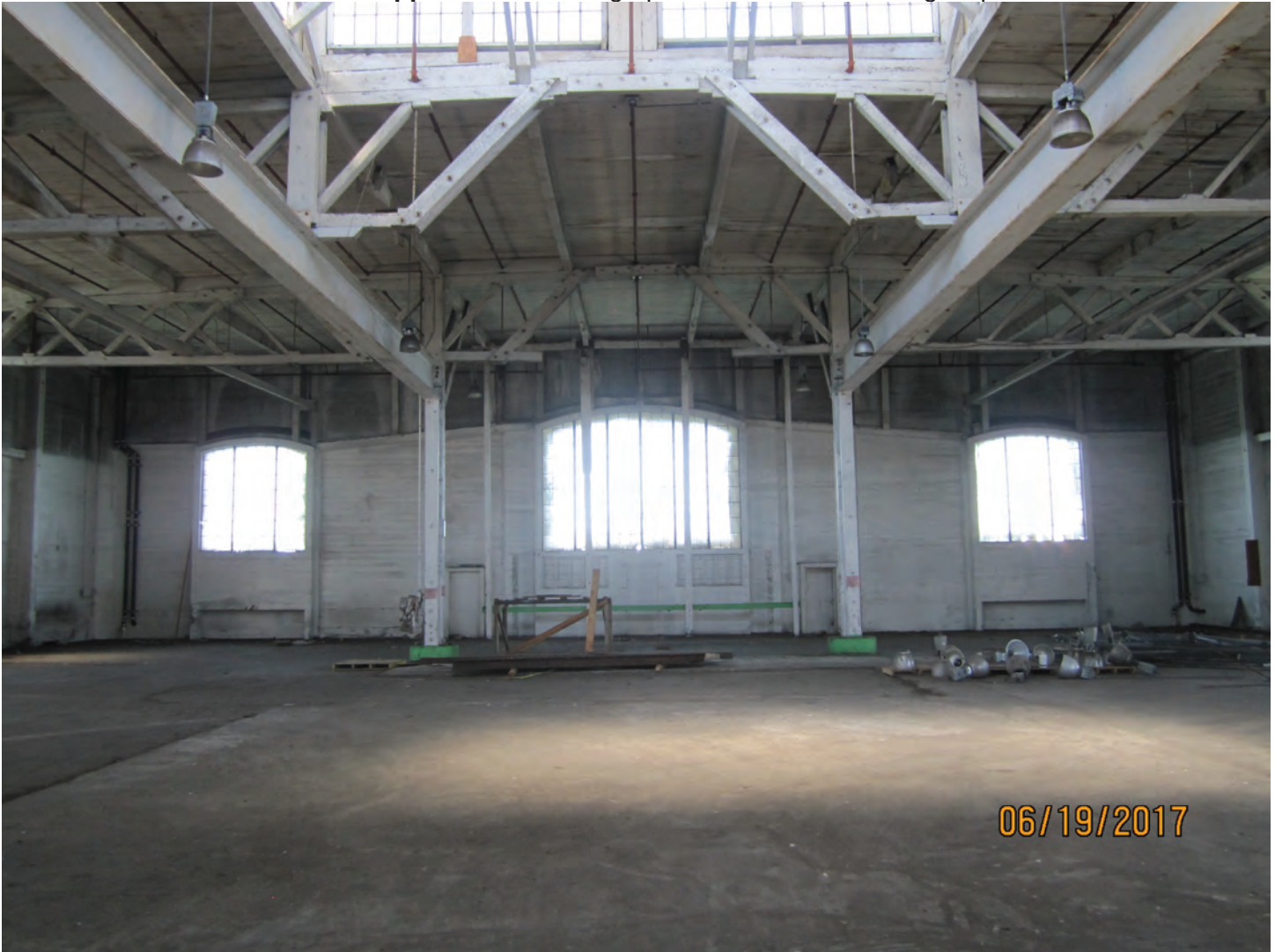
Photo 11. Rear concrete wall viewed from inside shed.
