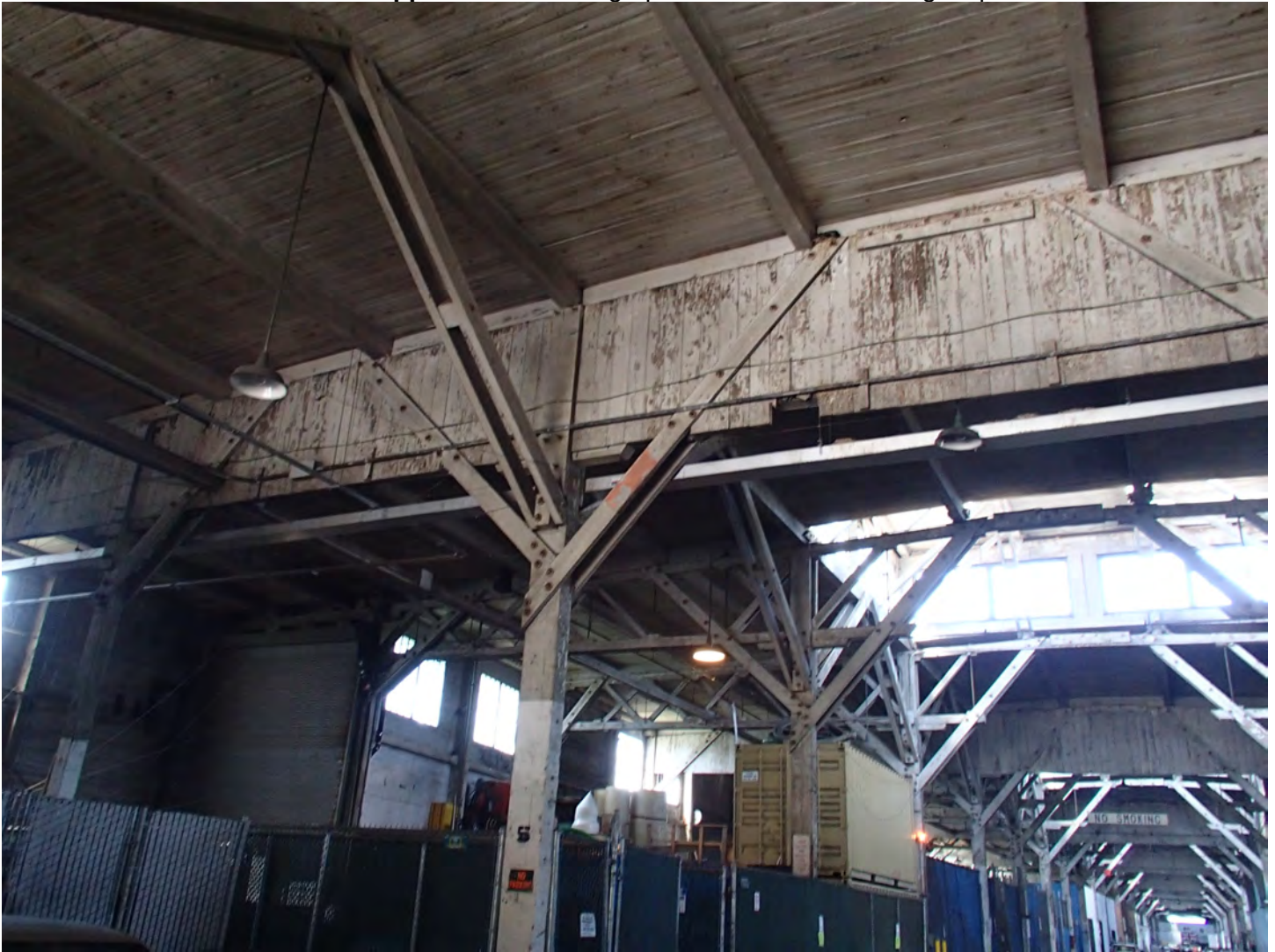
Photo 12. View of the interior timber column
