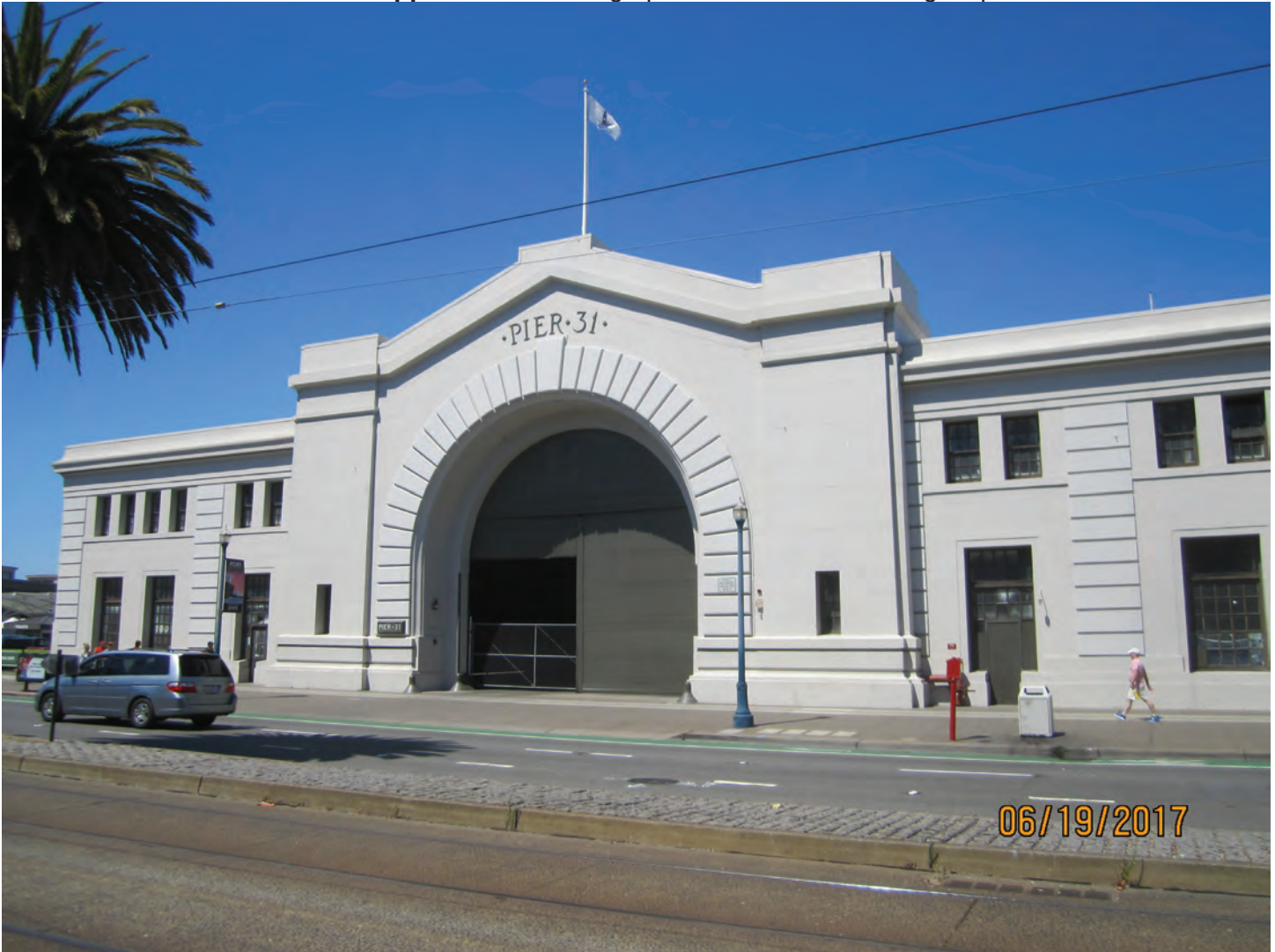
Photo 1. Bulkhead portion of Pier 31 shed building.
