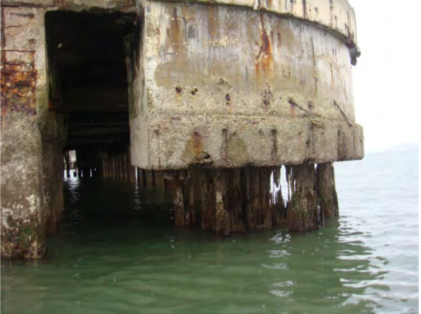
Photo 1. South wale piles seen from south apron
