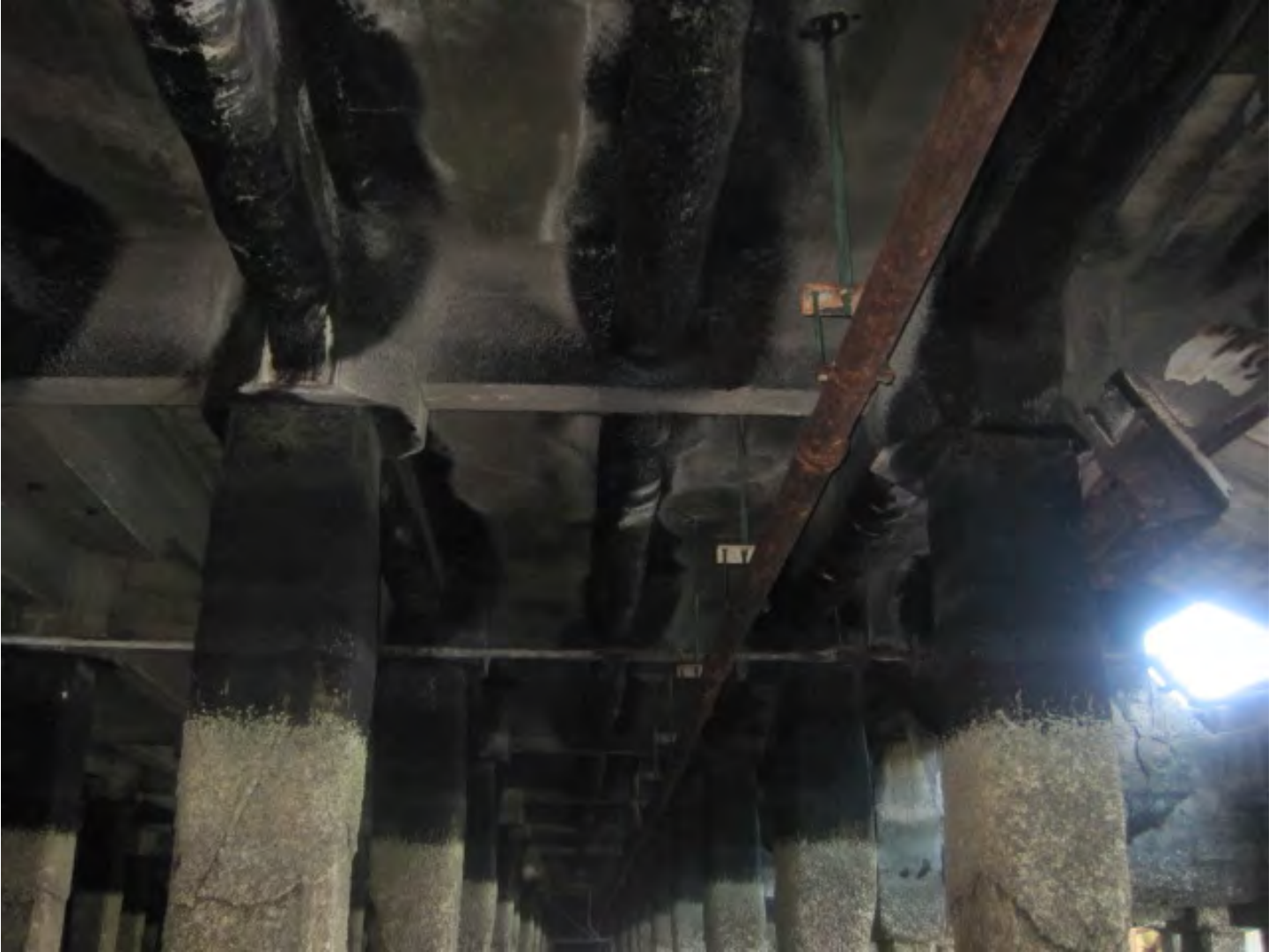
Photo 2. Gunite on concrete framing
