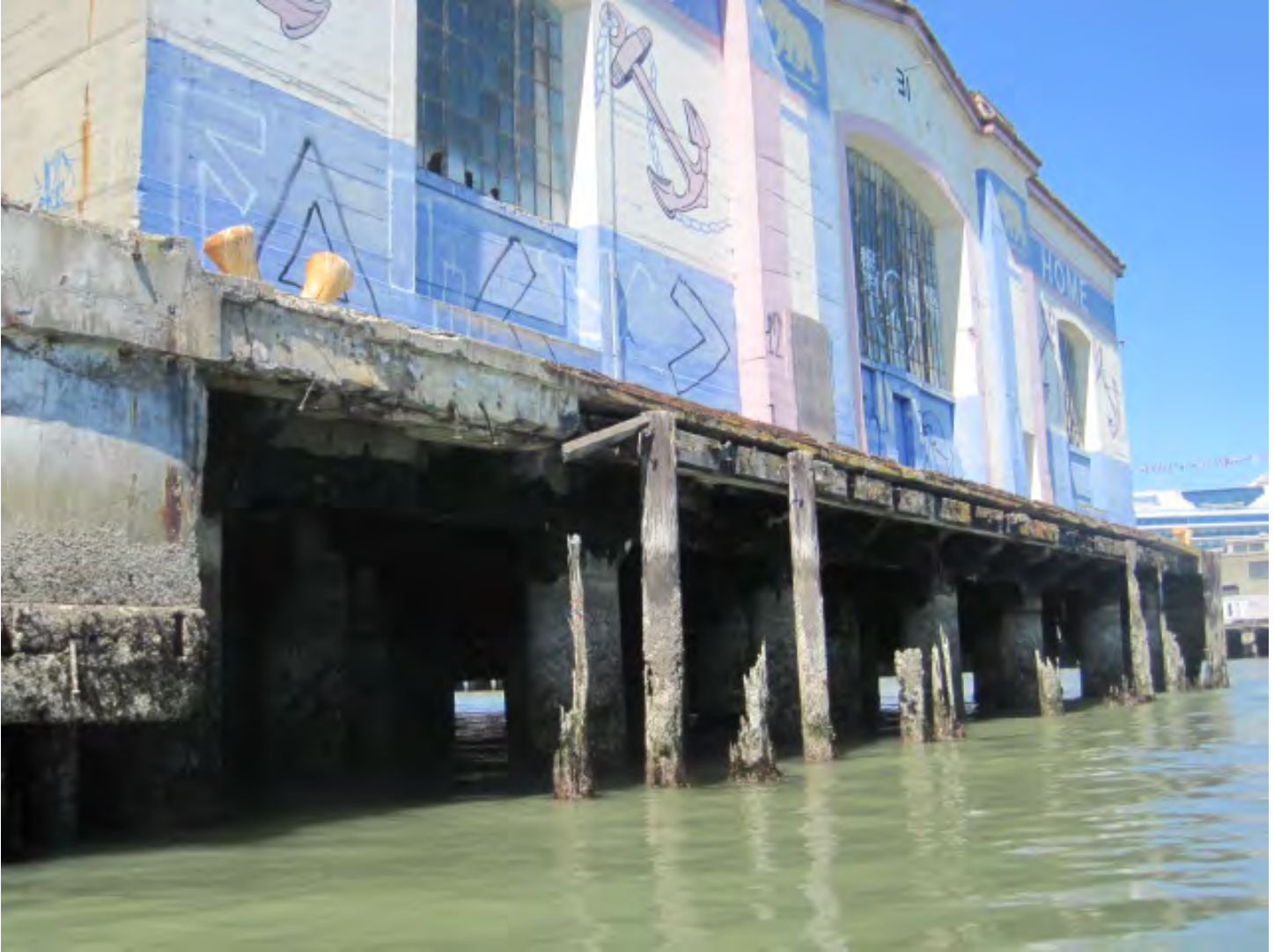
Photo 3. Overall view looking at east end
