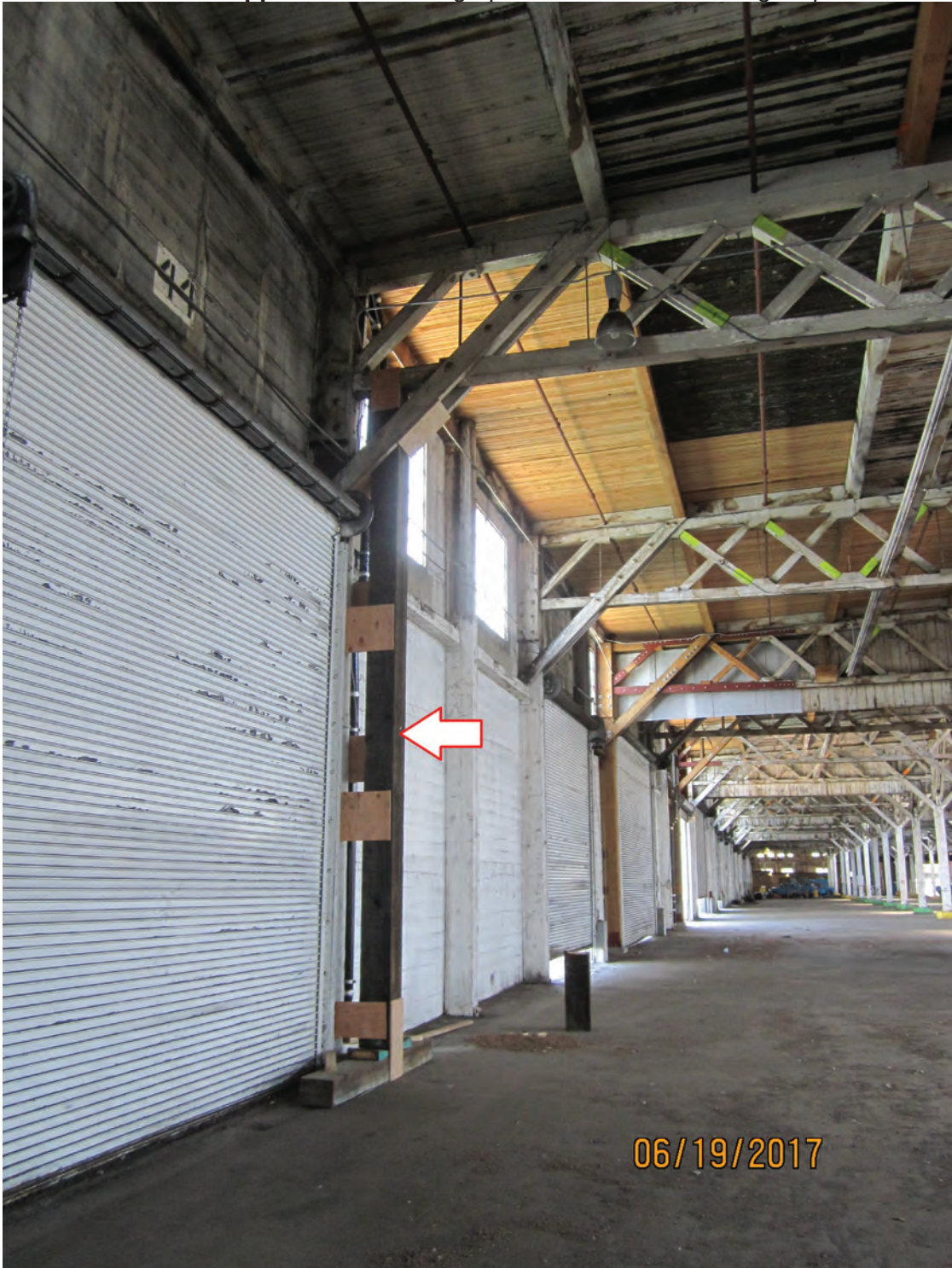
Photo 16. Shoring post installed at column grid H26 due to additional dry rot discovery. Permanent repairs are already planned. Similar shoring at B14 and B42. Roof area supported by these posts are shown yellow tagged until permanent repairs are complete.
