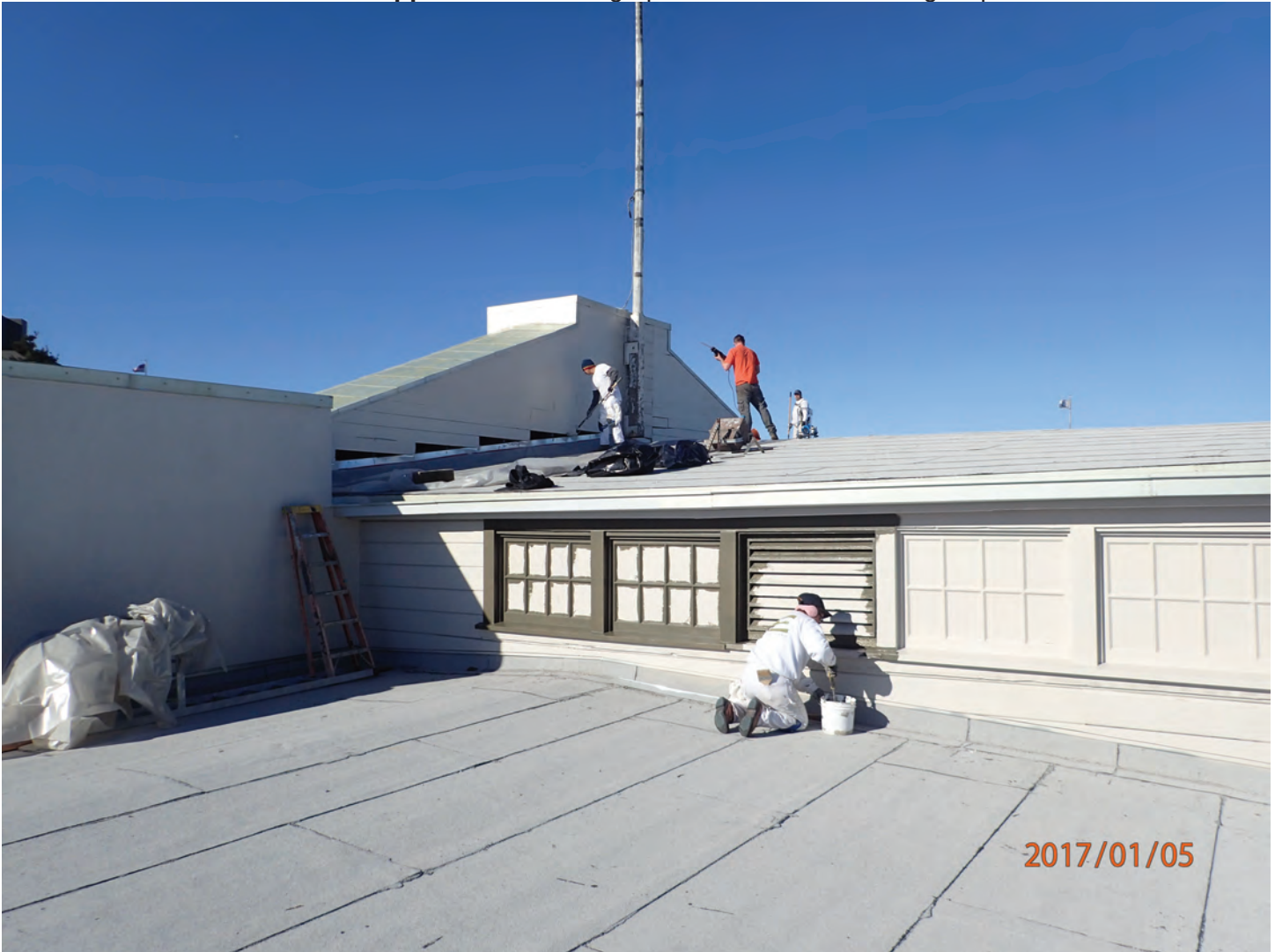
Photo 18. Construction photo of roofing work near bulkhead.
