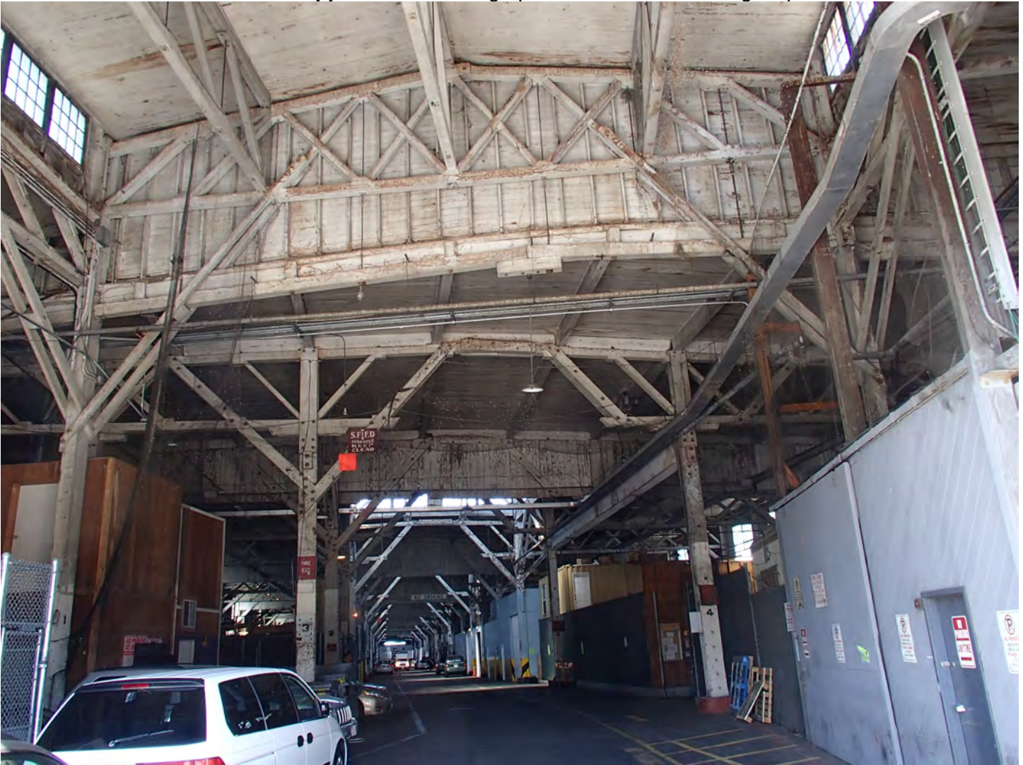
Photo 9. View of the structural framing near the interior entrance of the shed
