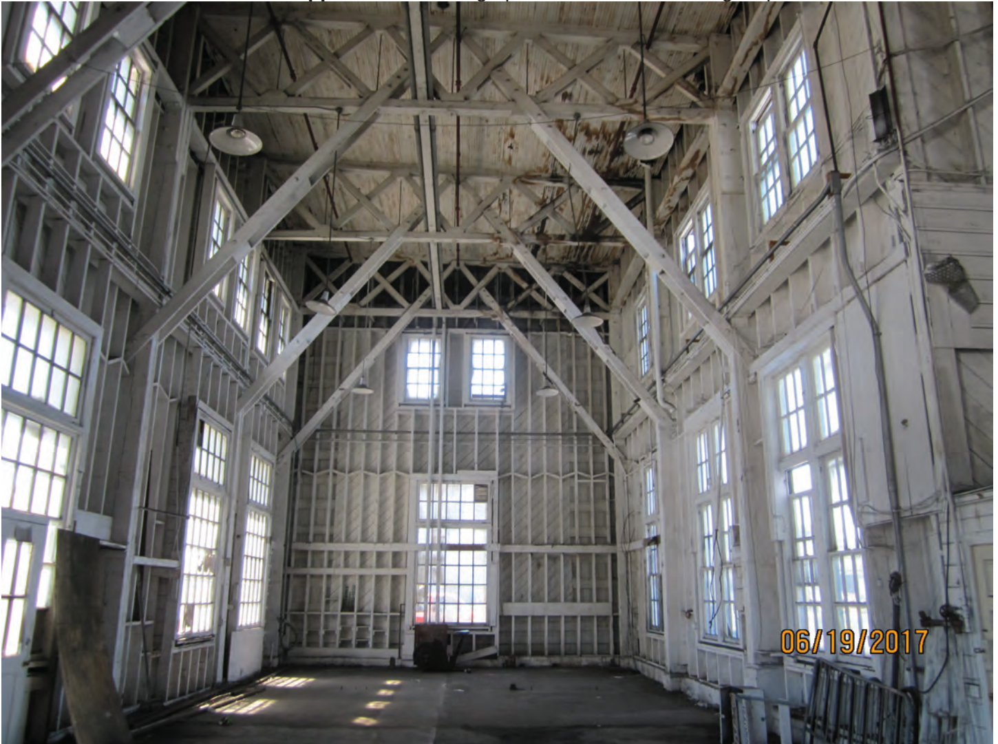
Photo 5. Typical bulkhead framing.
