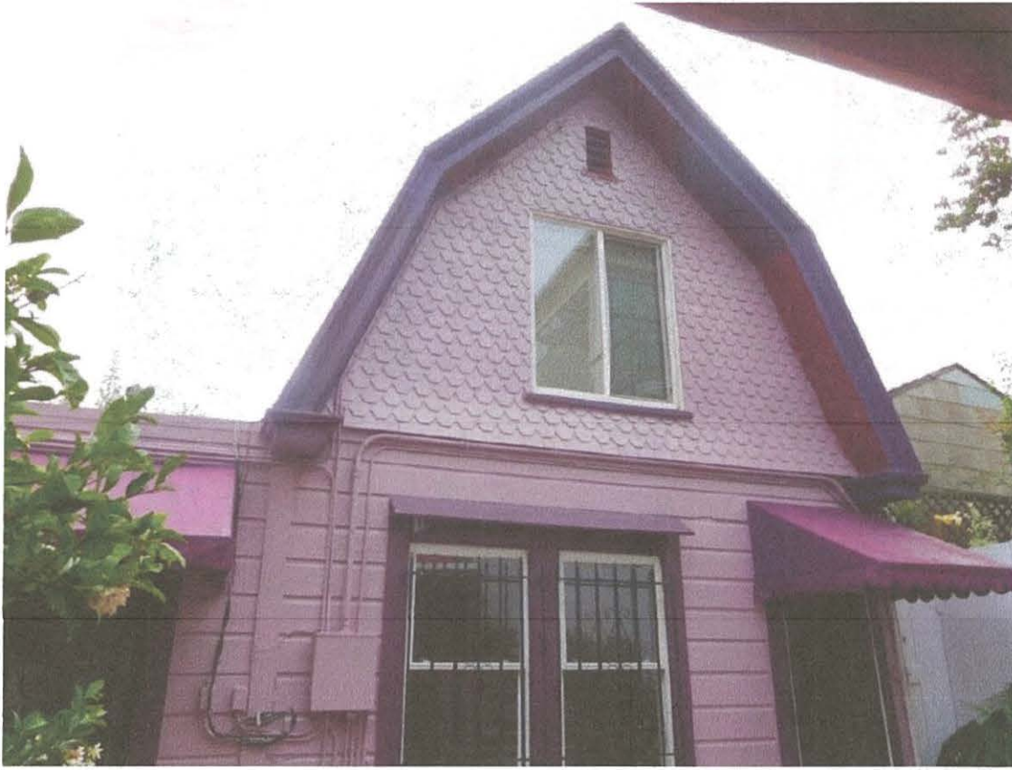
Figure 1. 617 Sanchez Street, residence building. Source: 617 Sanchez Street HRE.
