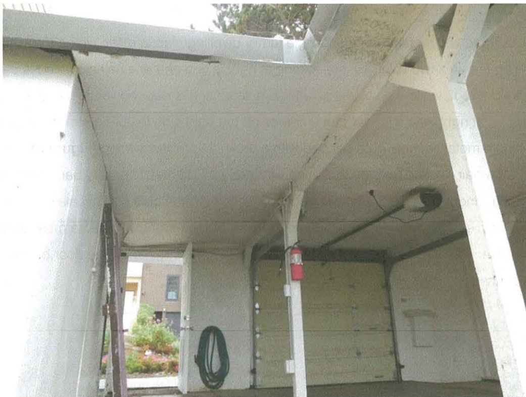
Figure 2: 617 Sanchez Street, front carport, interior
