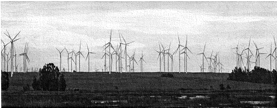
Photo 9: Shiloh I Wind Farm
