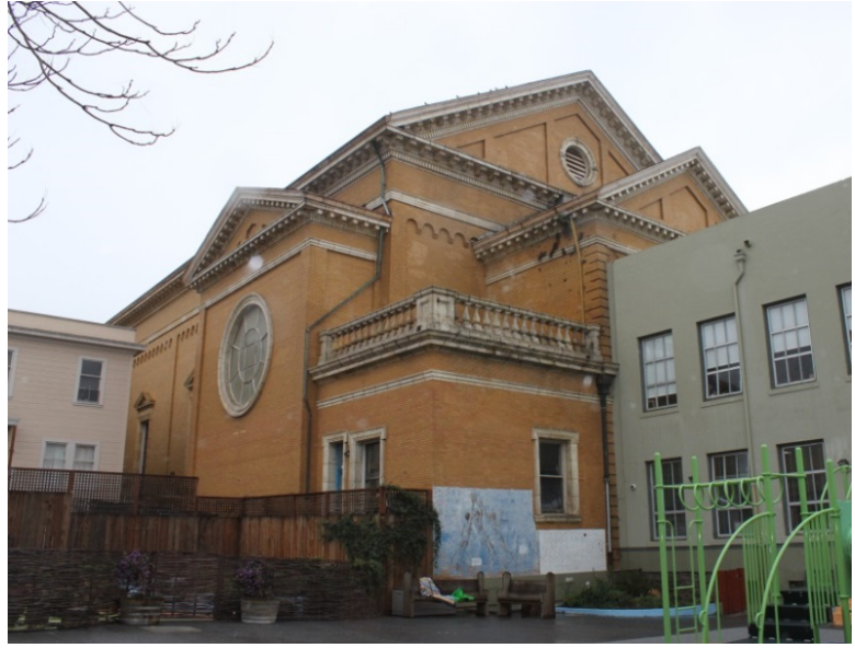
FIGURE 12. CHURCH: REAR, EAST ELEVATION FROM INTERIOR OF LOT, 2016.
