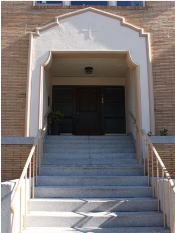
FIGURE 39 (LEFT). RECTORY: MAIN ENTRANCE, 2015.
