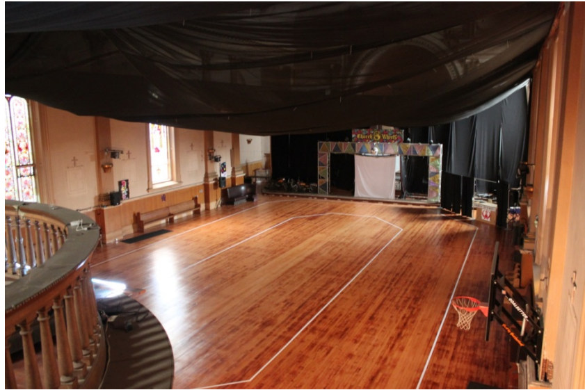
FIGURE 24: CHURCH: NAVE, LOOKING NORTHEAST FROM CHOIR LOFT, 2016.
