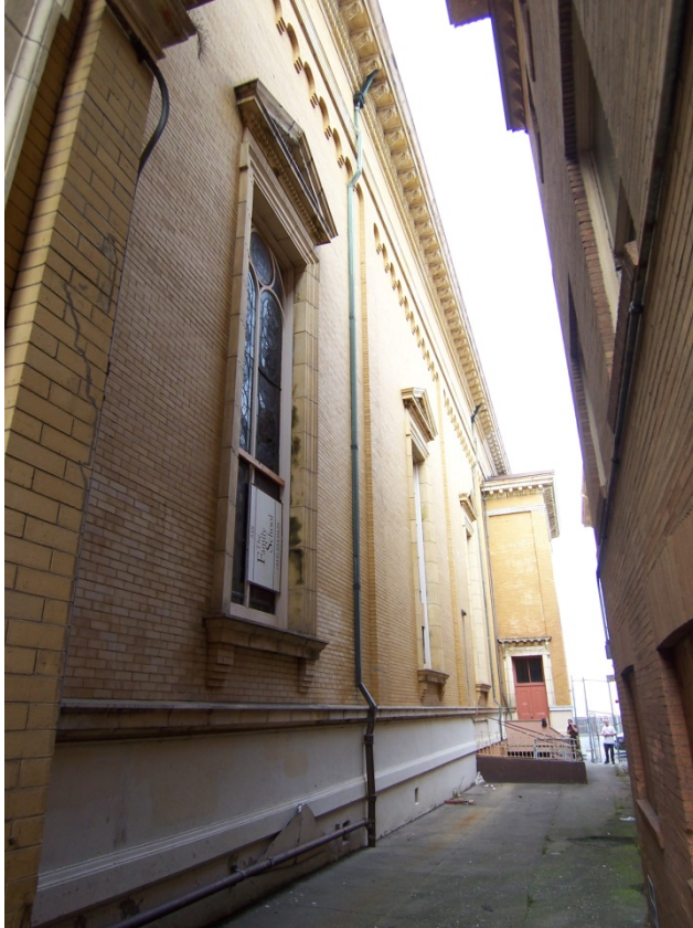
FIGURE 10. CHURCH: SOUTH ELEVATION LOOKING EAST. (PHOTO 2009. COURTESY CHRIS VERPLANCK)
