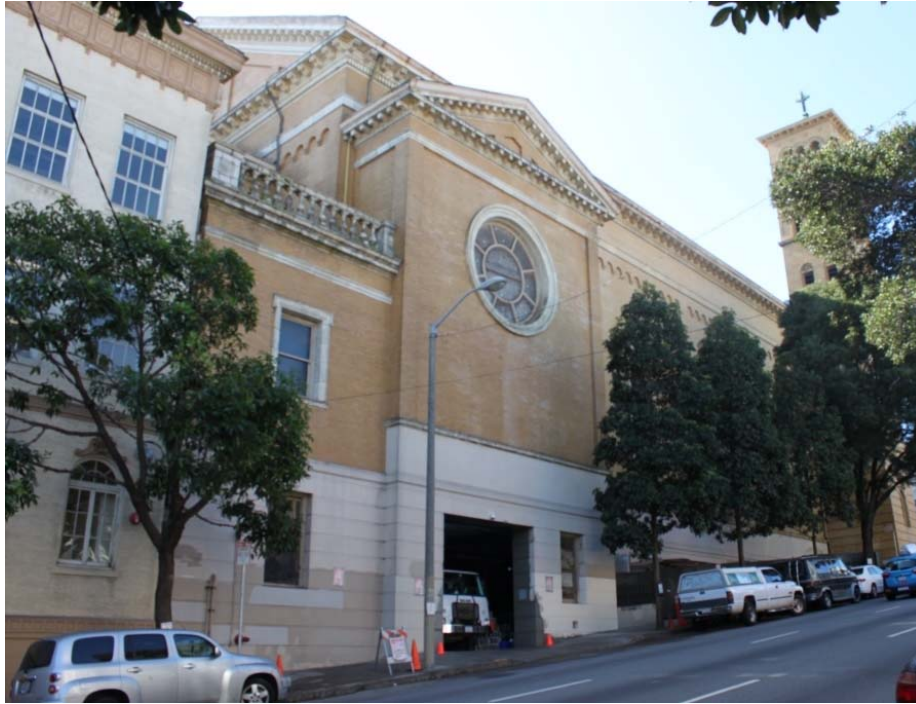
FIGURE 8. CHURCH: NORTH ELEVATION, LOOKING SOUTHWEST FROM FELL ST., 2015.
