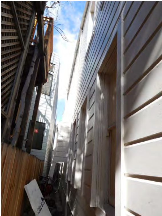
Figure 23. West façade; view toward north.
