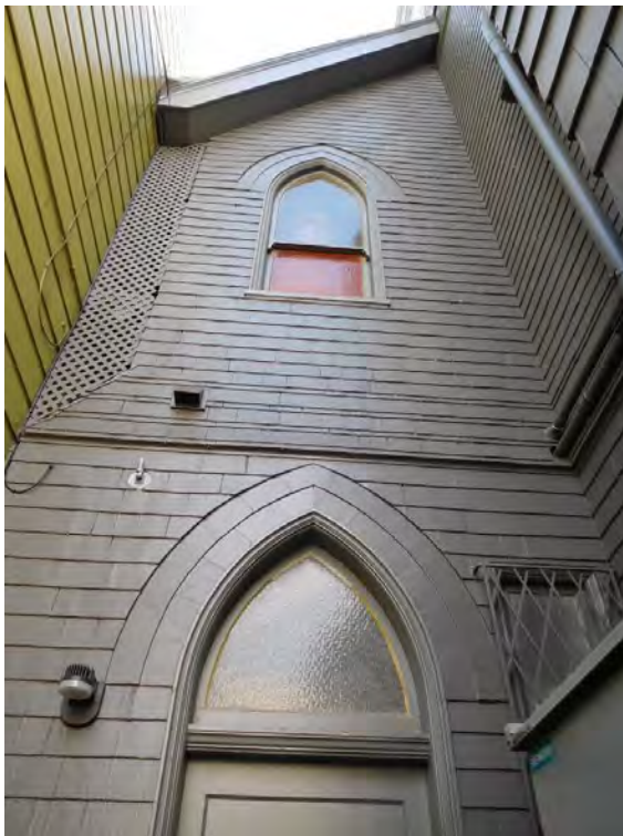
Figure 20. East transept; view toward south.
