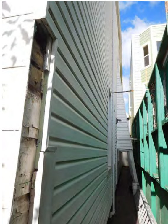
Figure 24. East façade; view toward north.
