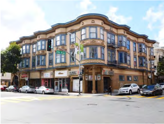
Figure 8. Classical Revival apartment building at southwest corner of 14 th and Valencia Streets; view toward southwest.
