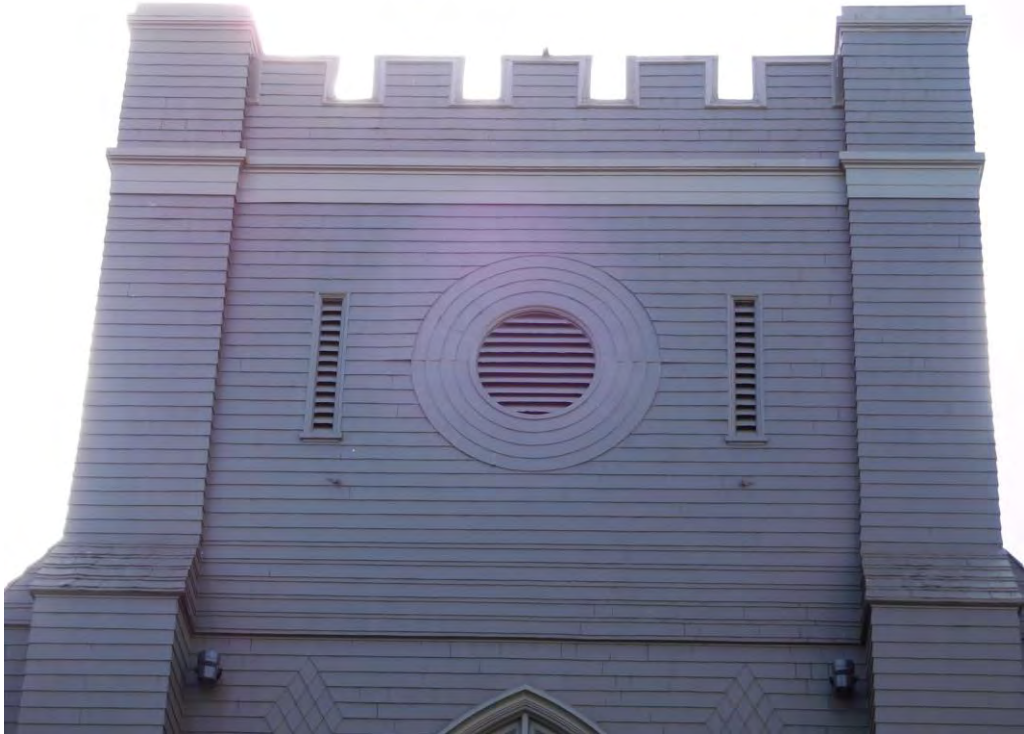
Figure 19. Belfry and parapet; view toward south.
