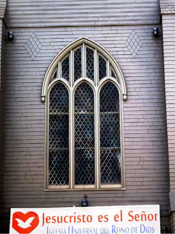
Figure 18. Gothic window on primary façade; view toward south.
