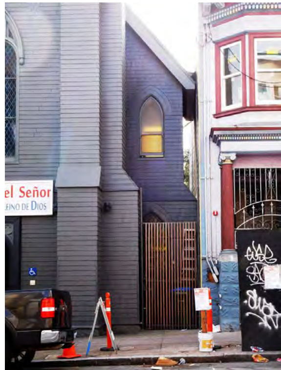
Figure 21. West transept; view toward south.
