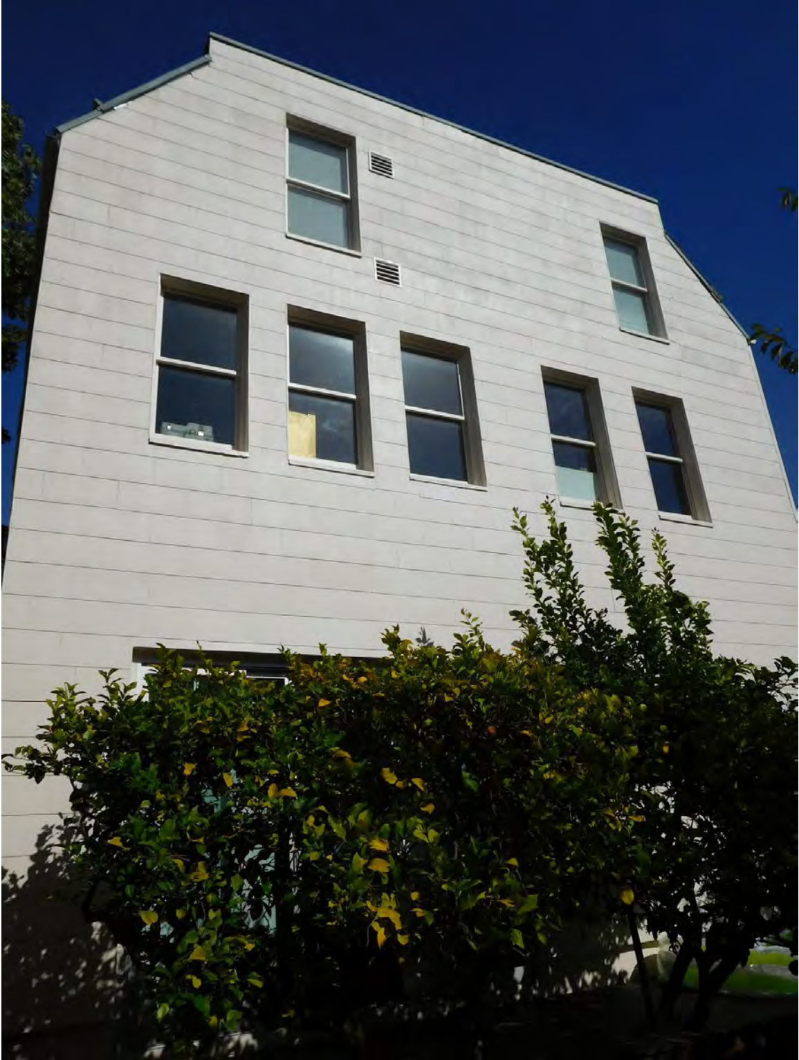
Figure 22. South façade; view toward north.
