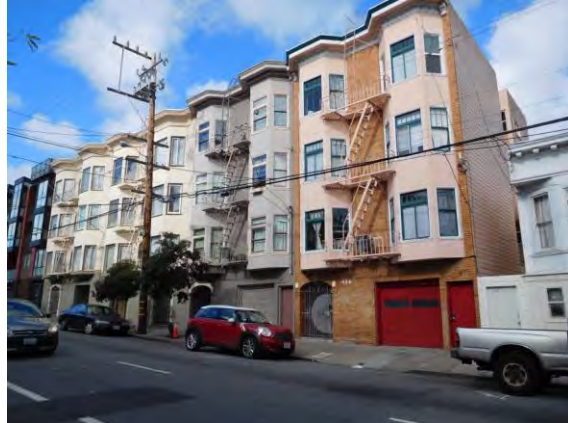
Figure 3. Renaissance/Baroque-style apartment buildings at 456 to 470 14 th Street; view toward northwest.
