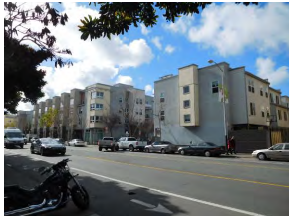
Figure 15. Valencia Gardens; view toward southwest from intersection of 14 th and Valencia Streets.
