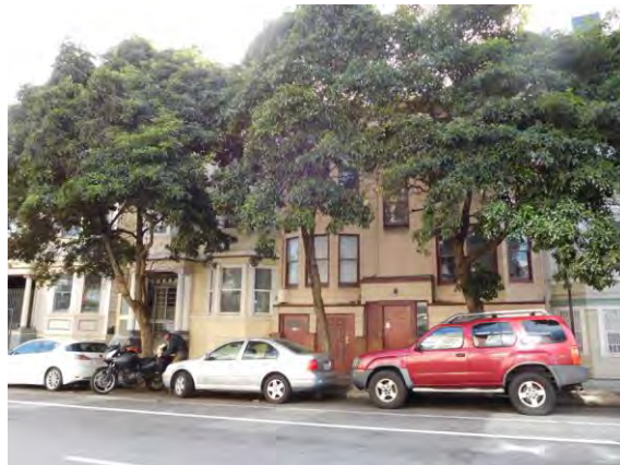
Figure 11. Romeo flats at 467-71 (left) and 477-81 (right) 14 th Street; view toward south.
