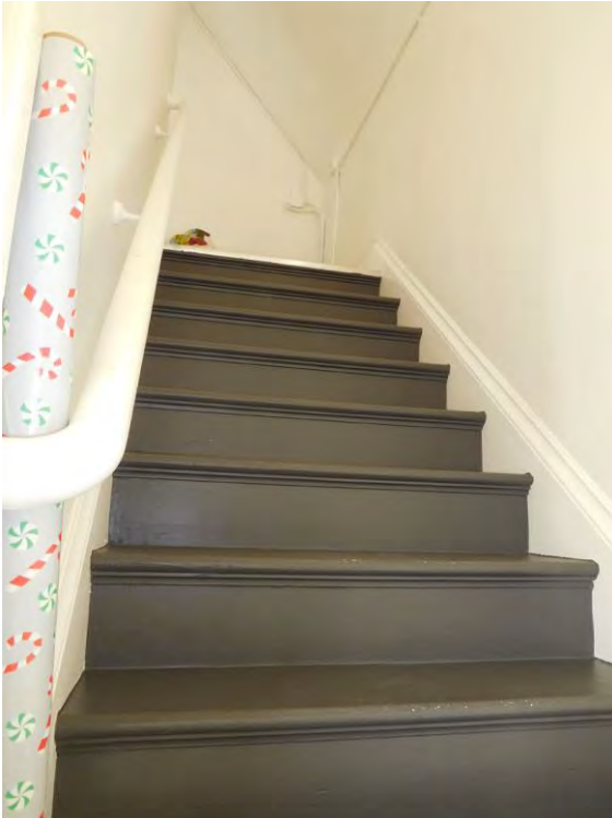
Figure 40. Stair leading to third floor; view toward north.
