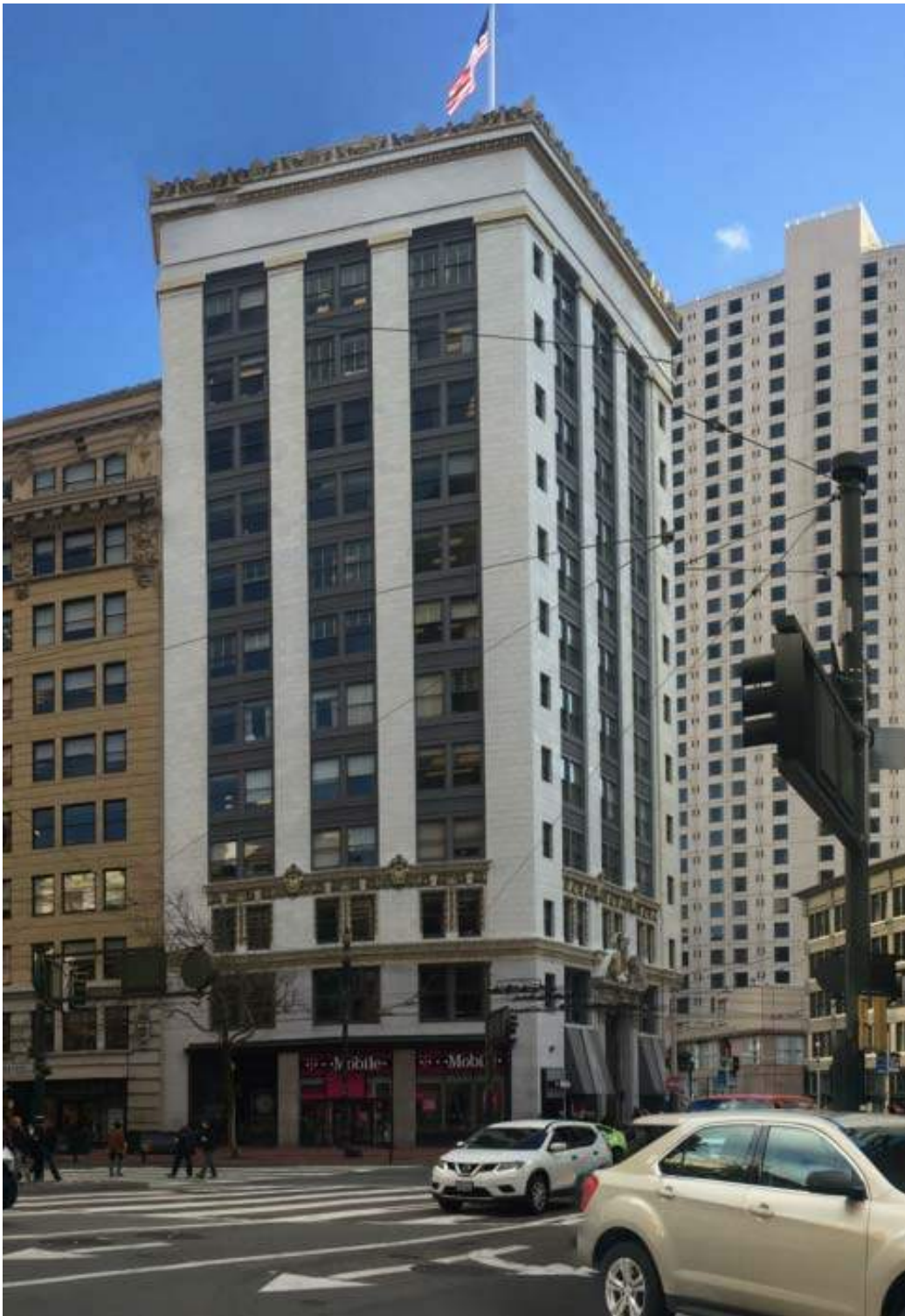
EXISTING view looking southeast from Market Street
