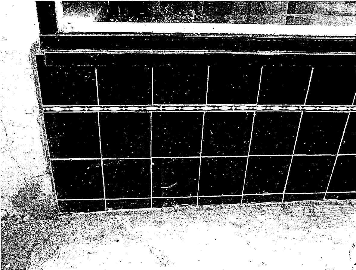
Figure 5 Black tile bulkhead with lozenge and bead narrow course as seen here at the east end of 198 Gough Street's commercial facade on Oak Street.
