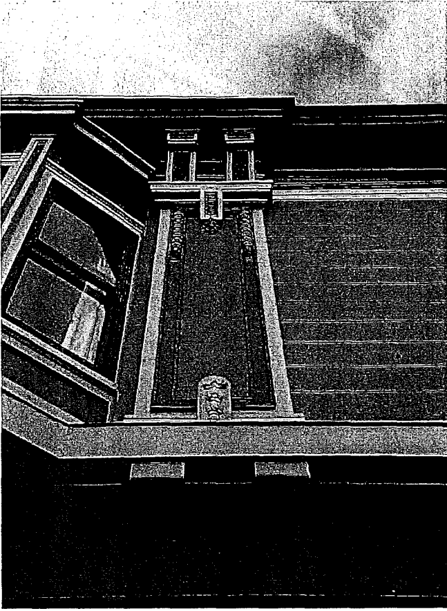
Figure 3 Classical elements from the Beaux Arts palette including the measured use of moldings to create crisp cornice and panel elements create an impression of exceptional refinement and design quality to R. L. Goldberg Building's edifice.
