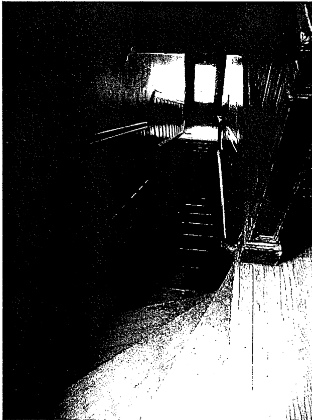
Figure 30 High ceiling in the commercial units on the first floor require a high stairwell from the front doors to the flats of the Goldbergs' residences. Pictured is Rube Goldberg's entry stairs with original woodwork and lath and plaster.
