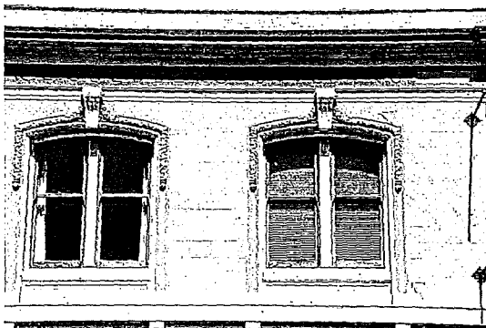
R. L. Goldberg Building, 182-198 Gough Street
