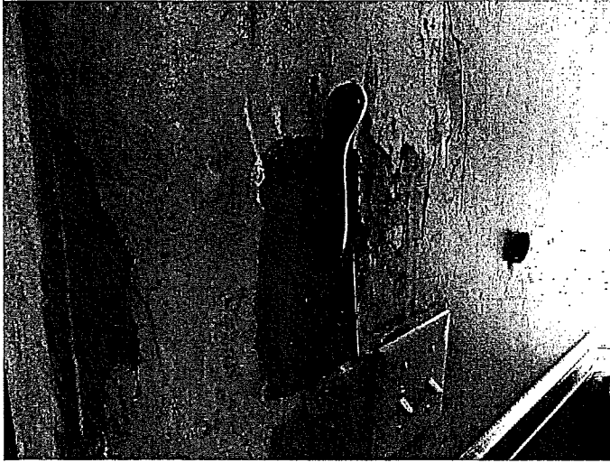
Figure 29 The bronze handle and speaking-horn at the top of the stairwell at 194 Gough Street is unlike Rube Goldberg's elaborate machinations that accomplished a mundane task with great effort. These devices allowed him to communicate with the person at the front door downstairs and to pull the lever to open the door if they are welcomed guests without having to descend the steps himself.
