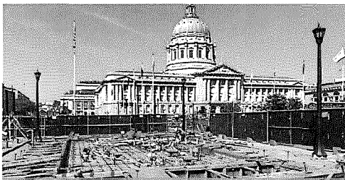
Bi-Rite Café Construction Begins
