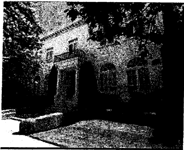
Comp 3 100 Commonwealth Ave
