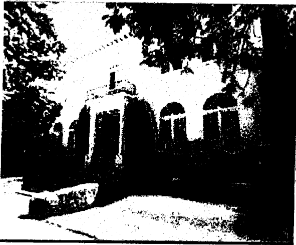
Comp 3 100 Commonwealth Ave
